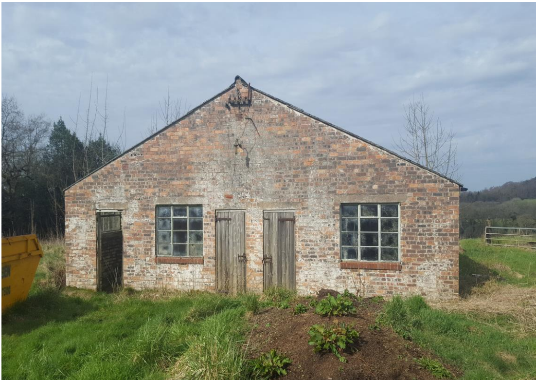
General view of gable elevation
