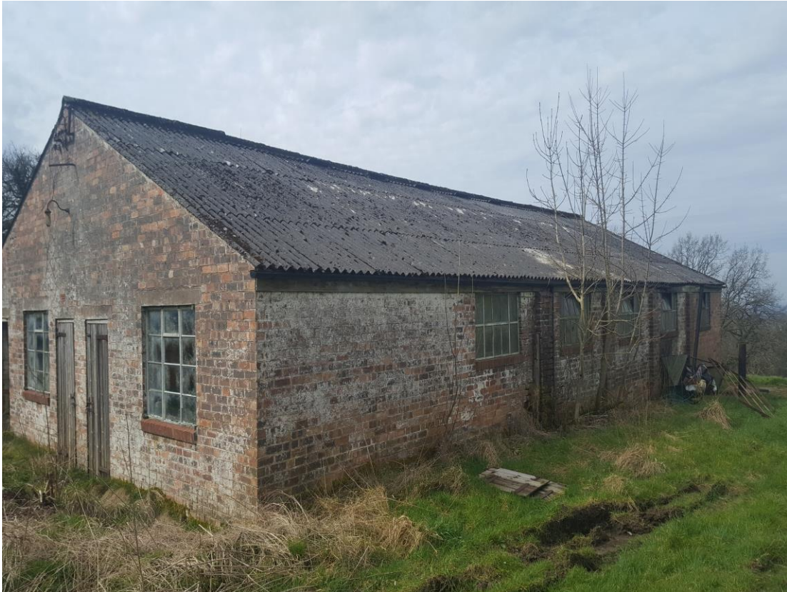
General view of side elevation of barn
