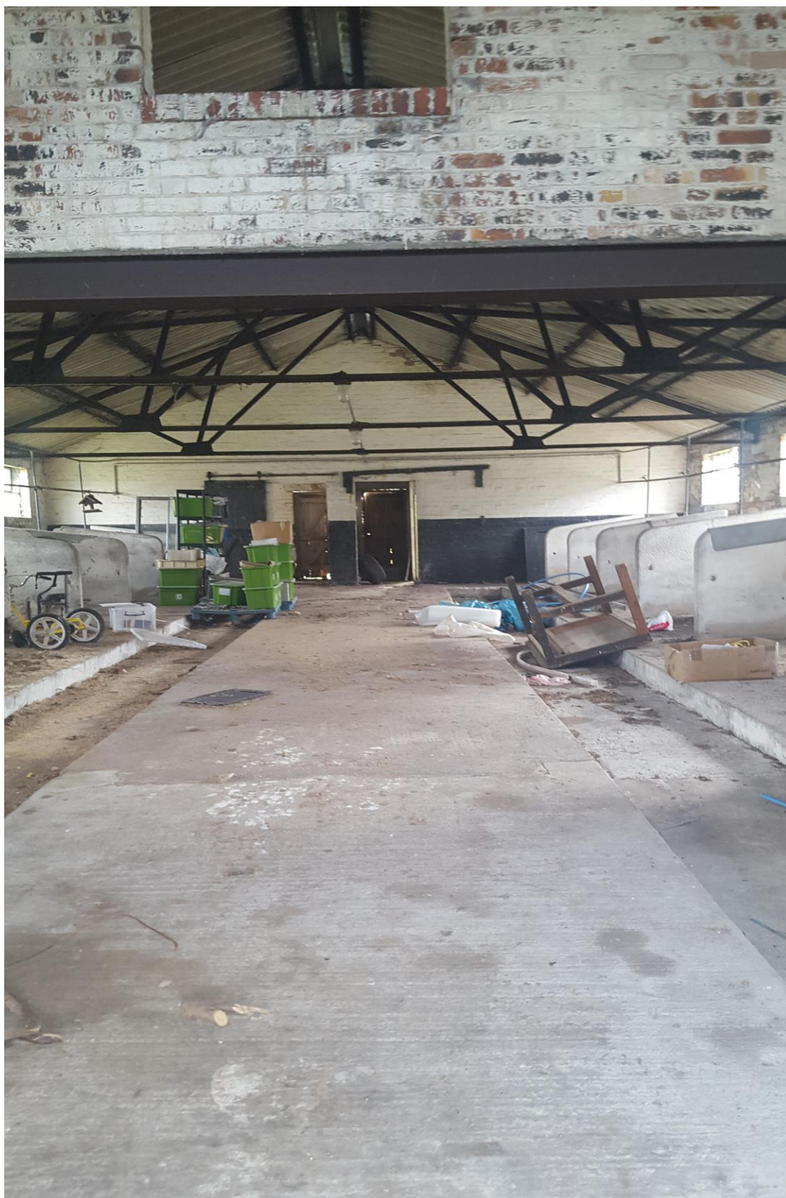
General internal view.
