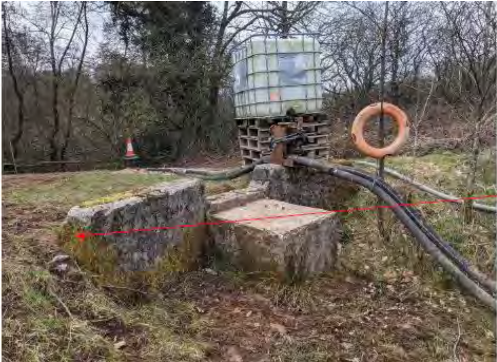
Figure 8-6: Outlet weir structure (adapted from Mott MacDonald (2021))
