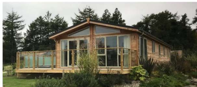
Typical Pitched Horizontal Timber Clad Lodge. Pale Grey Powder Coated Aluminium Frames. Galvanised Rainwater Goods. Pressed Metal Roof. Timber Skirt and Deck Posts
