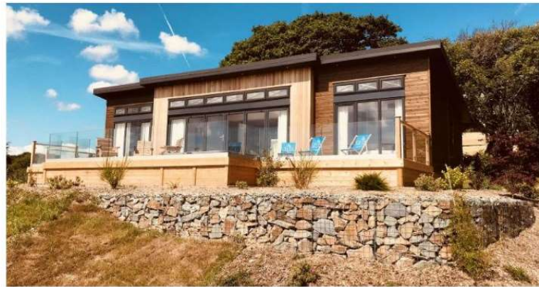
Typical Monopitch Timber (Vertical & Horizontal) Clad Lodge. Pale Grey Powder Coated Aluminium Frames. Galvanised Rainwater Goods. Pressed Metal roof. Timber Skirt and Deck Posts
