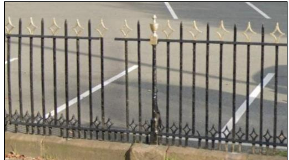
Railings on Congleton Road, © 2022 Google, image taken Oct 2021
