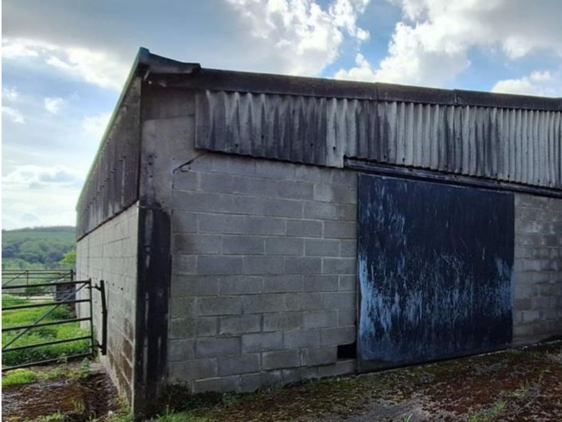
Plate 23: Image showing the eastern elevation of B5.
