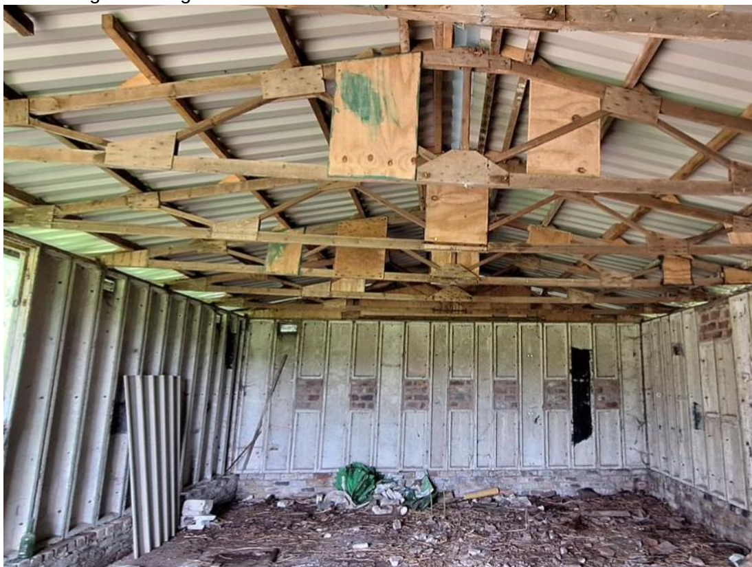
Plate 34: Image showing the internal of B7 .
