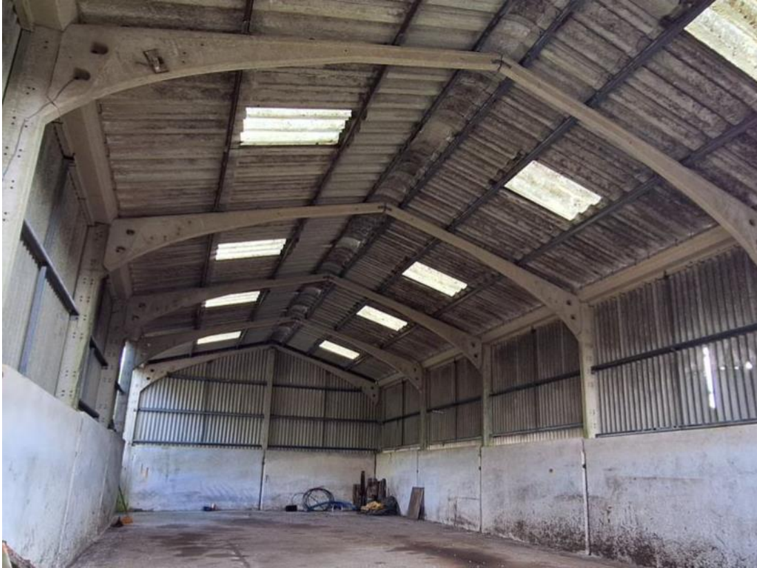
Plate 29: Image showing the internal of B6.
