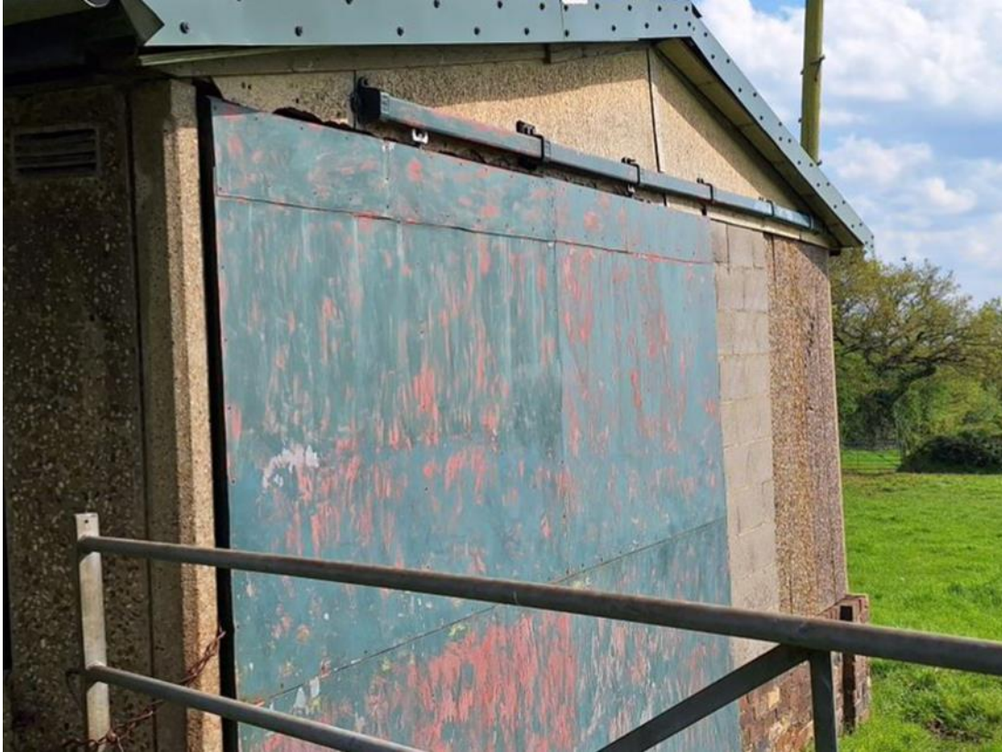
Plate 31: Image showing the eastern elevation of B7.
