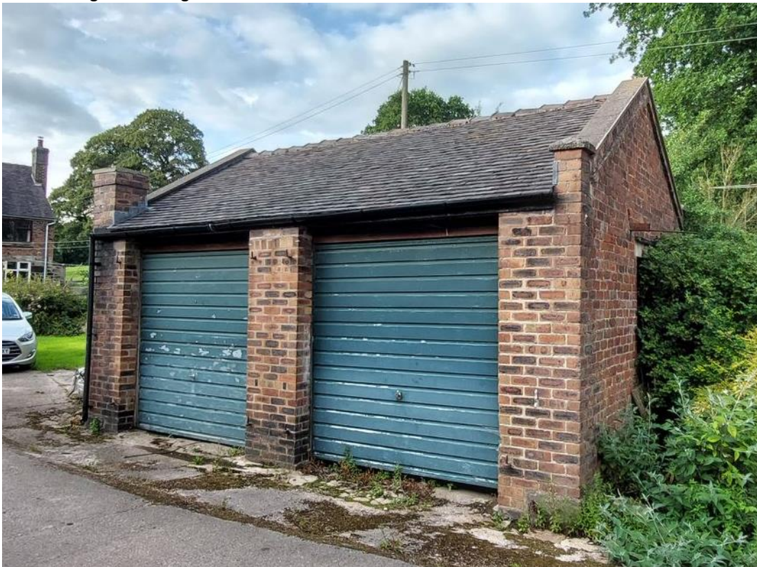
Plate 18: Image showing the eastern and southern elevation of B3.
