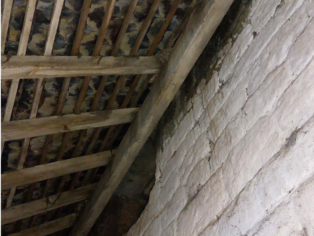
Plate 17: Image showing interior of the southern extension of B2.
