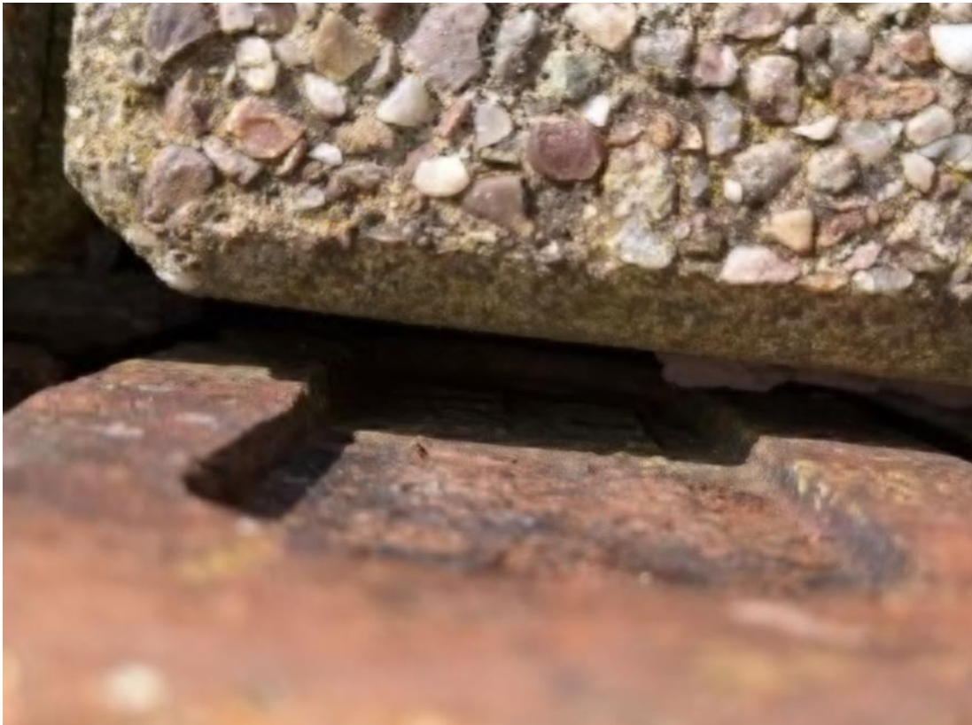
Plate 32: Image showing the gap between the pebbledash rendering and the brick walls of B7.
