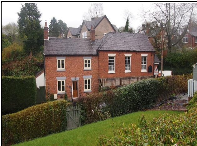
Plate 1: Chapel House and Methodist Chapel
