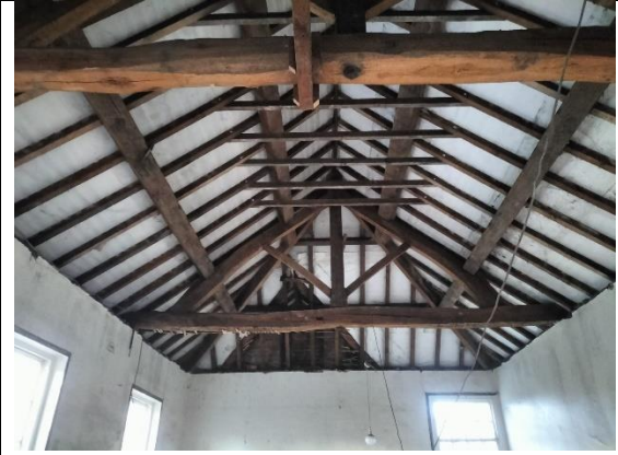
Plate 9: Exposed roof timbers
