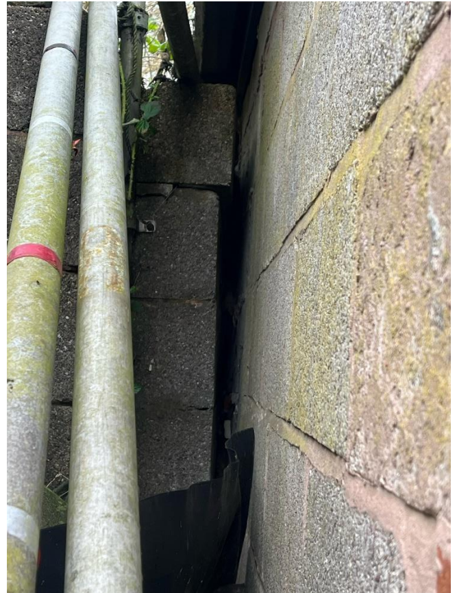
Image 2 Zoomed in rear of garage to be demolished and retaining wall for land at rear of 133 and 135 Station Road.
