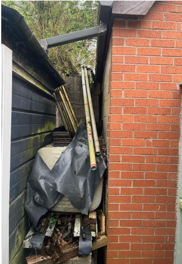
Image 1 Rear of garage to be demolished and retaining wall for land at rear of 133 and 135 Station Road.
