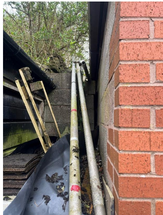
Image 3 Rear of garage to be demolished and retaining wall for land at rear of 133 and 135 Station Road.
