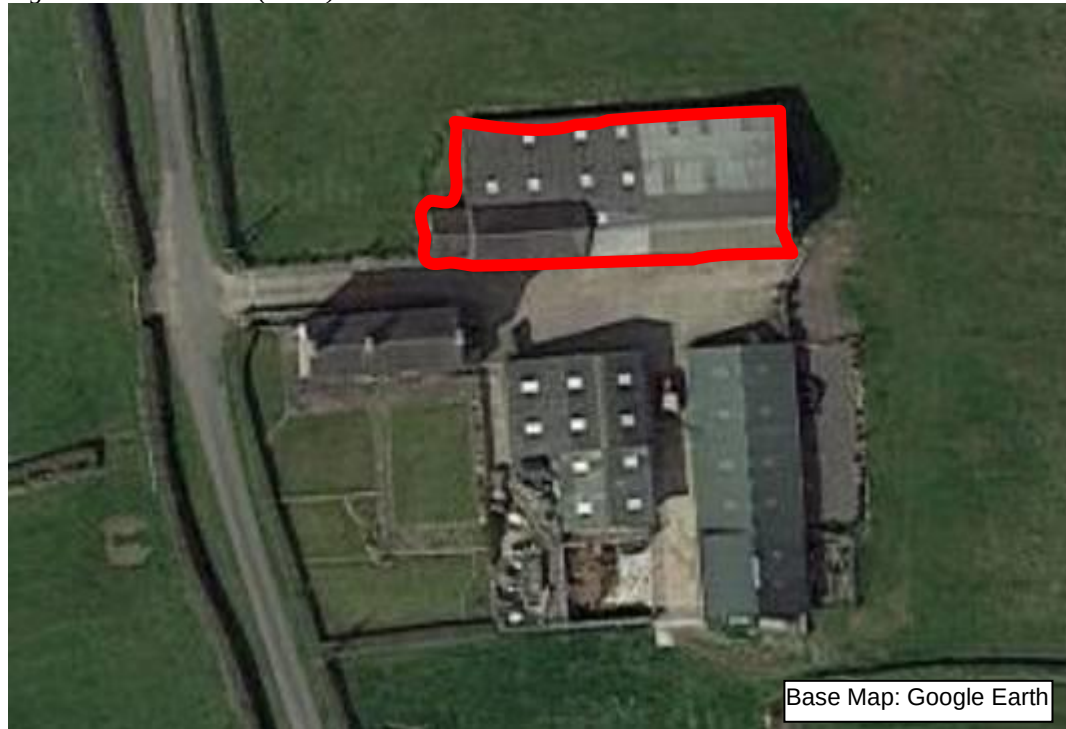
Figure A.3: Site Aerial (detail).
