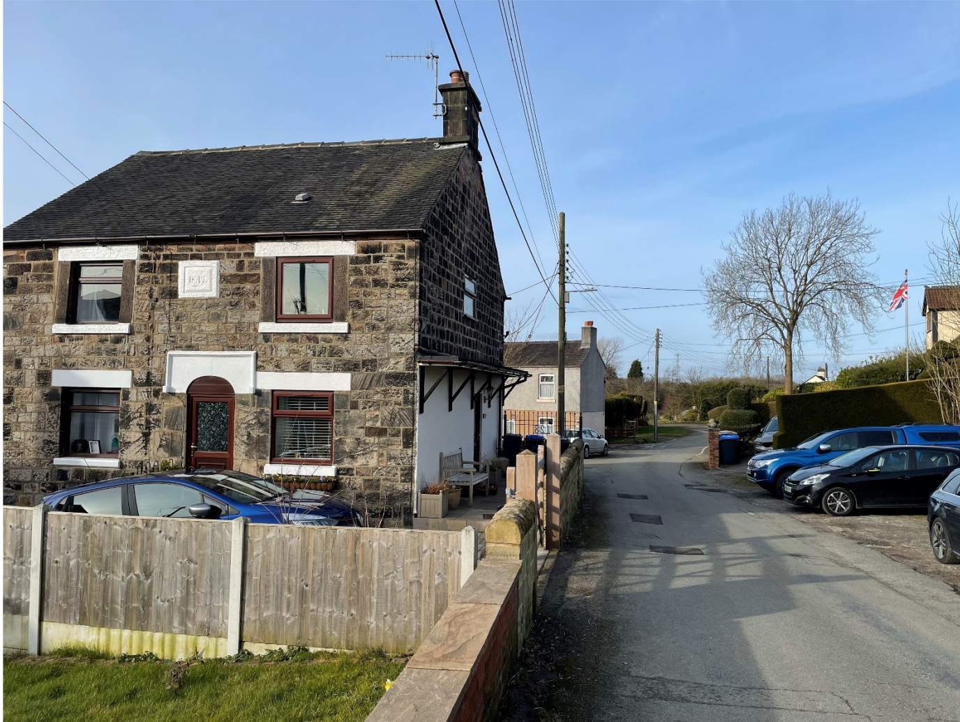
VIEW LOOKING NORTHWEST ALONG WASHERWALL LANE
