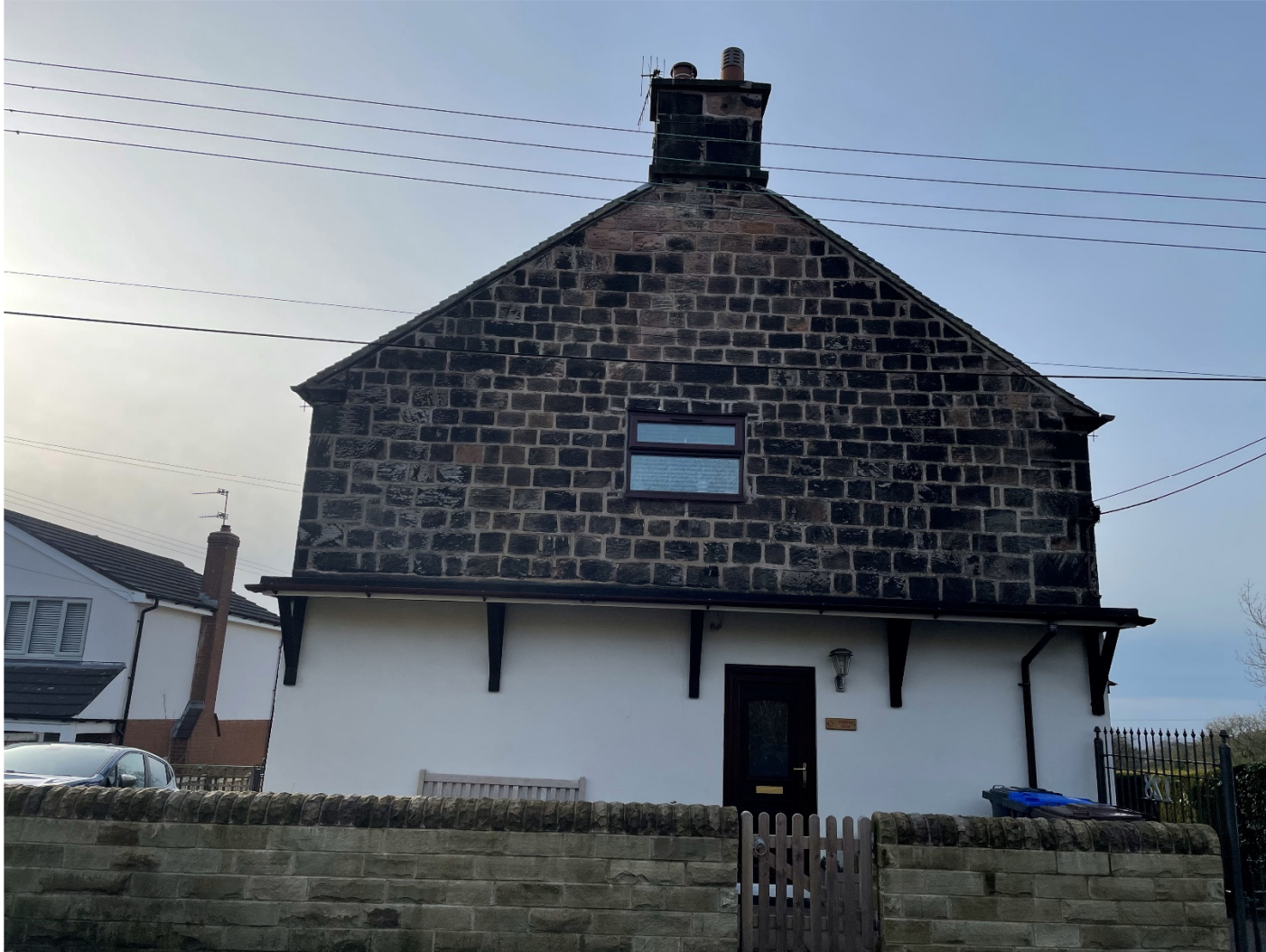
VIEW OF GABLE WALL FROM WASHERWALL LANE
