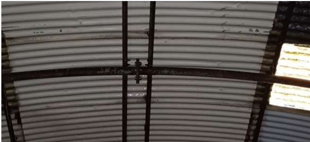
Figure 1 – Joint in steel frame
