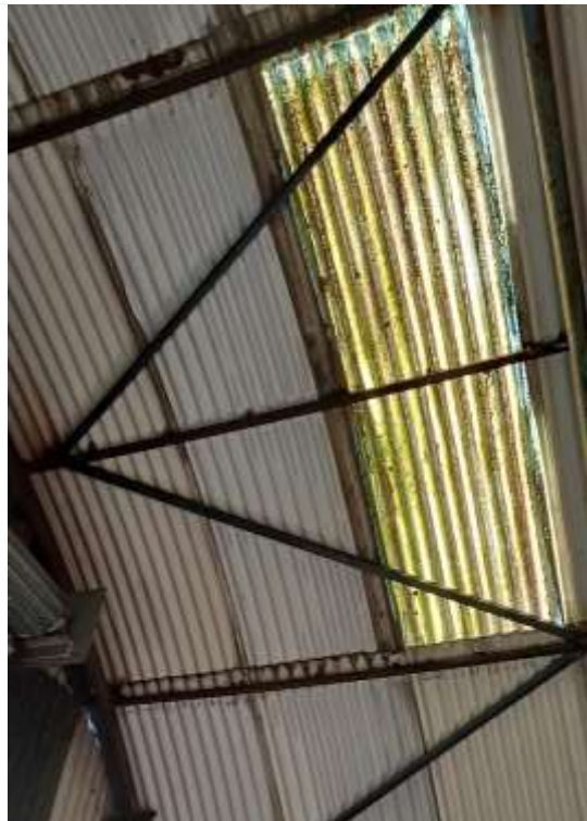
Figure 10 – Bracing to left side
