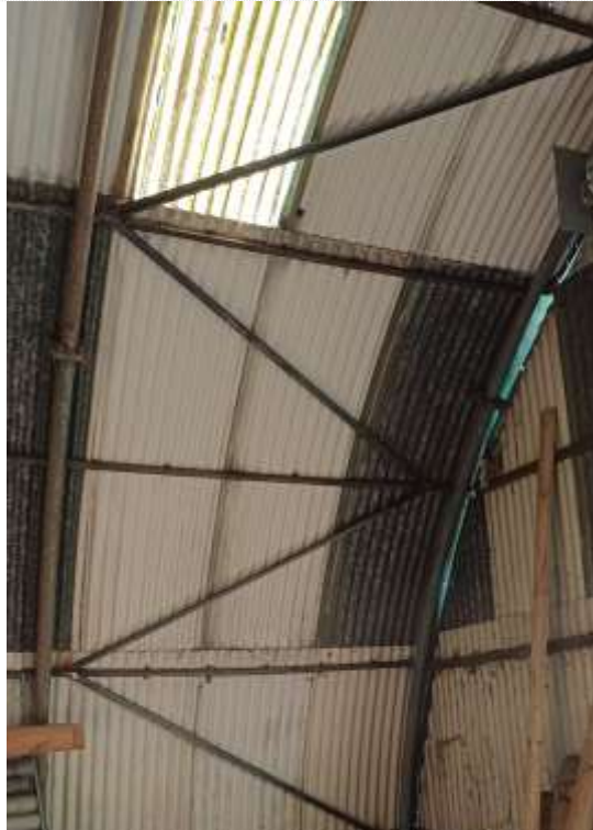
Figure 9 – Bracing to right side
