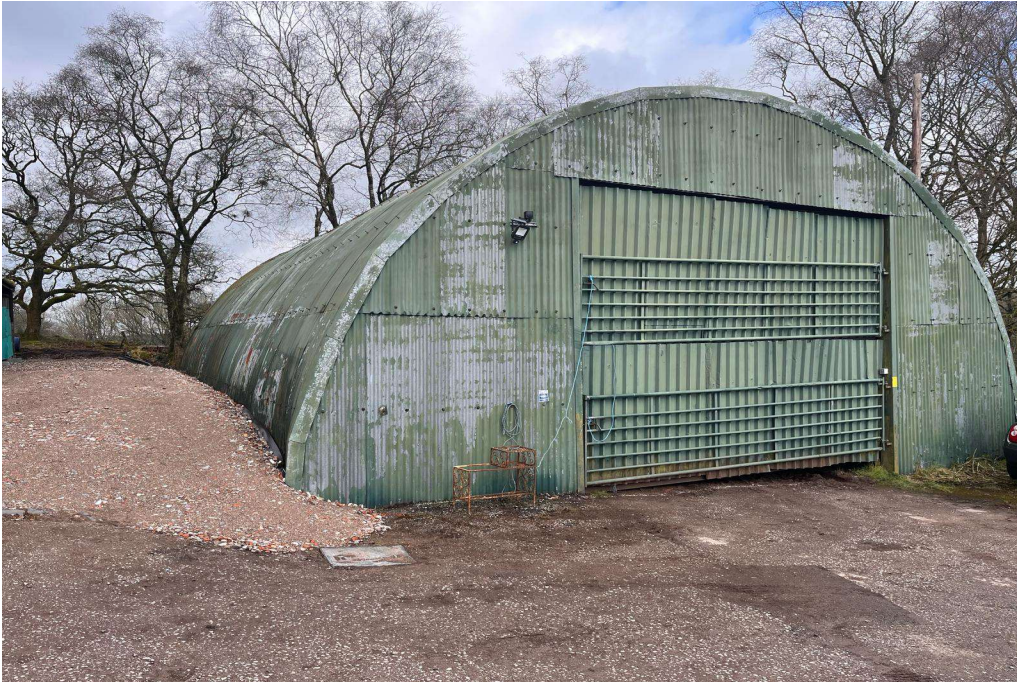
Existing building – South Elevation
