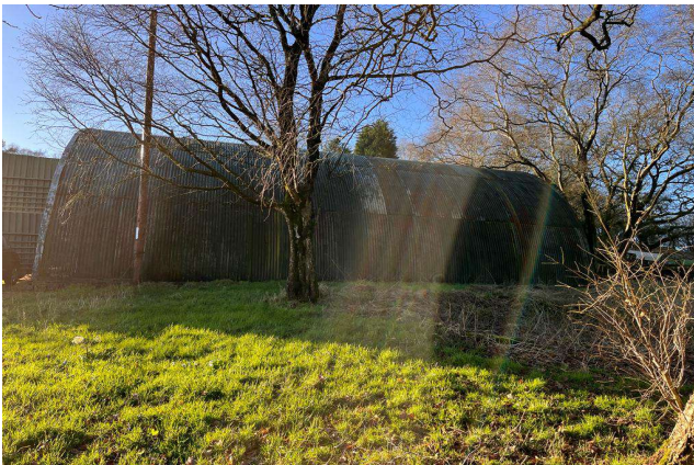
Existing building – East Elevation Facing Dial Lane
