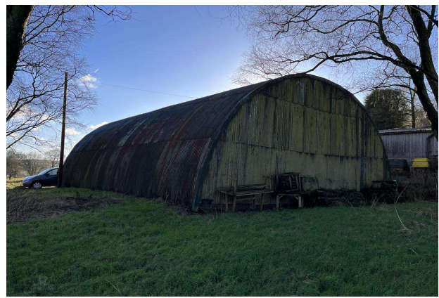
Existing building – North East Corner Rear
