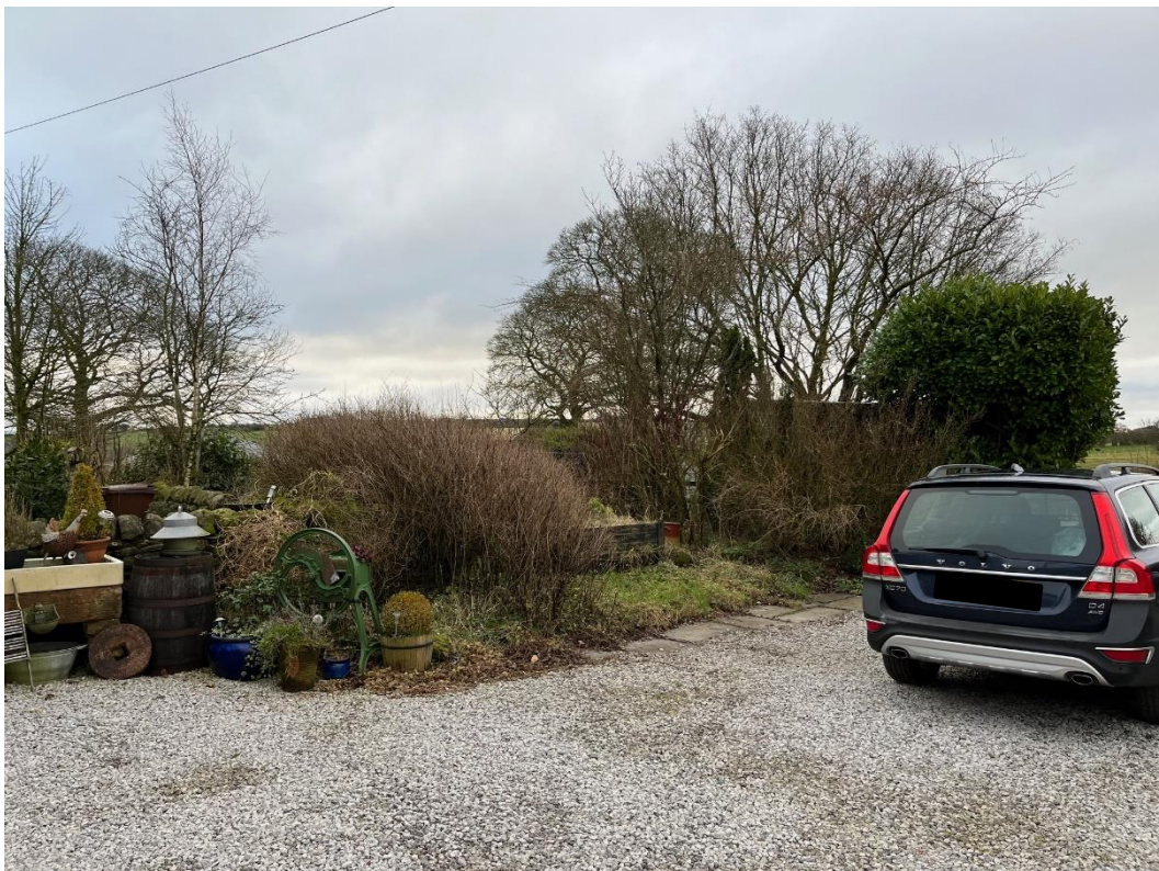
2. Site for new garage and existing driveway / parking
