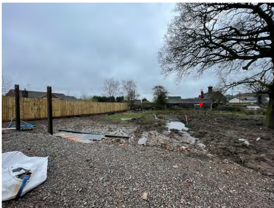
Plate 7. The outbuilding along to the northeast of the PDA.
