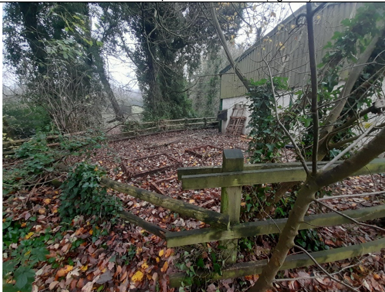
North elevation of the Visitor's Centre/fenced garden area (Figure 3)
