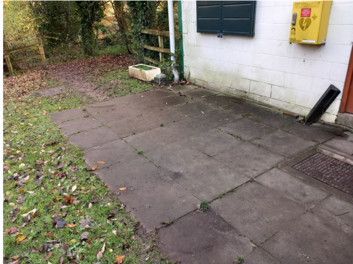
West elevation of the Visitor's Centre (Figure 2)
