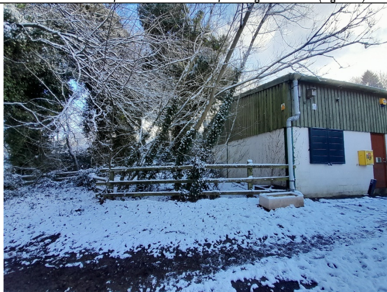
North/west elevations of the Visitor's Centre/fenced garden area (Figure 4)
