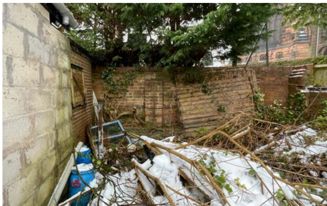
Existing brick boundary.
