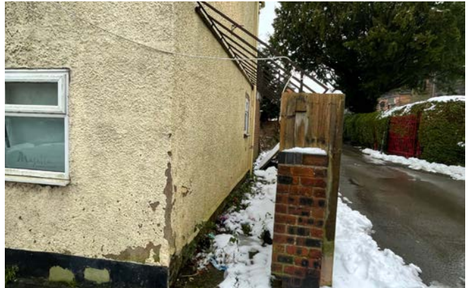
Existing side boundary.
