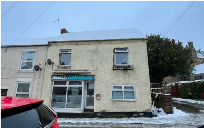
Existing front of building to be made good. All commercial signage to be removed.
