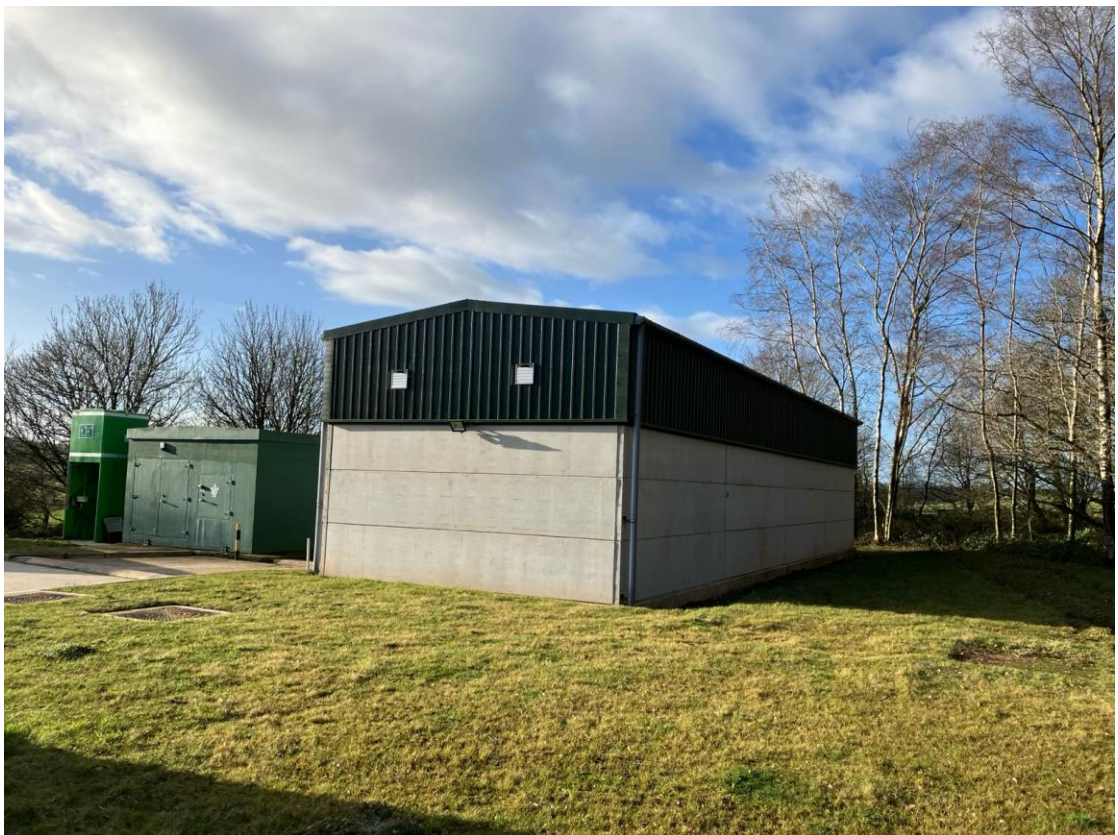
Figure 3 - Filtration Building (South-East Elevation)
