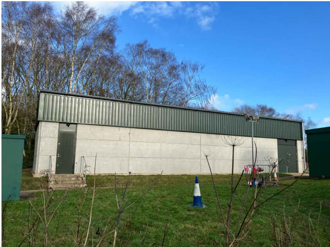
Figure 1 - Filtration Building (South-West Elevation)
