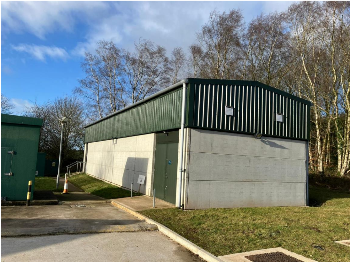
Figure 2 - Filtration Building (South-East Elevation)
