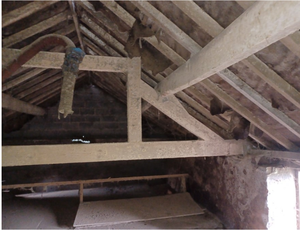
Photo 8: First floor showing the roof construction
