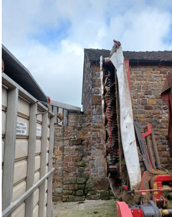
Photo 1: Front elevation showing the side gable with the cattle shed.
