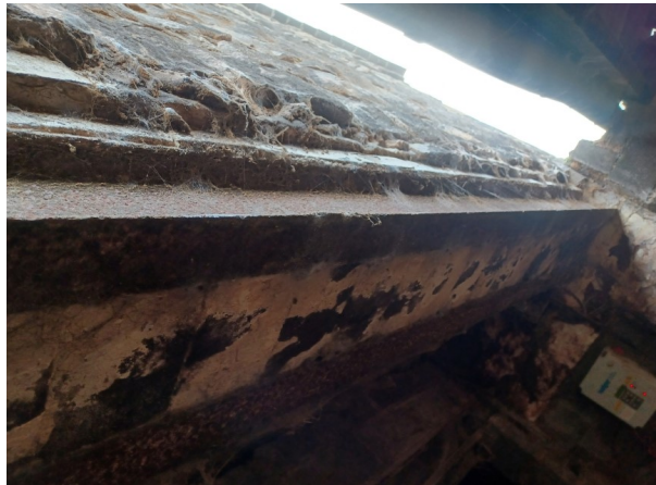
Photo 6: Gable wall with cattle shed showing steel supports
