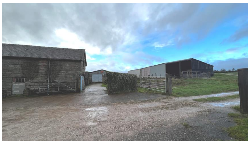
Fig 9. Looking West, Showing the access Track to the farm, barn east elevation and 2No modern farm buildings (photo: ctd architects 2023)
