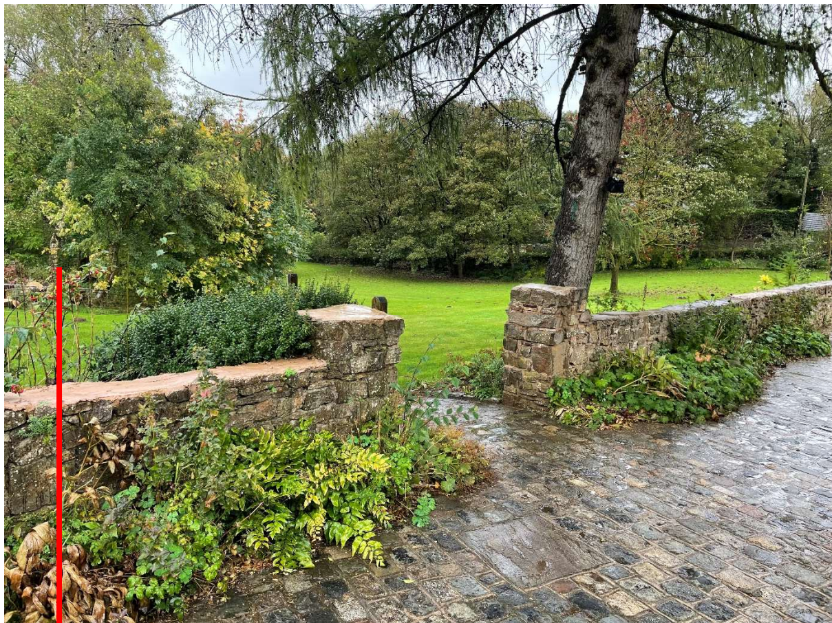
Stone pillar to be rebuilt in new position giving wider access.
