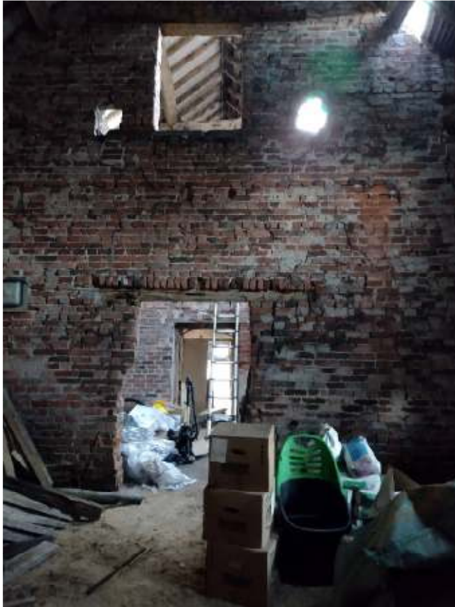
Photographic Plate 5: Internal view
