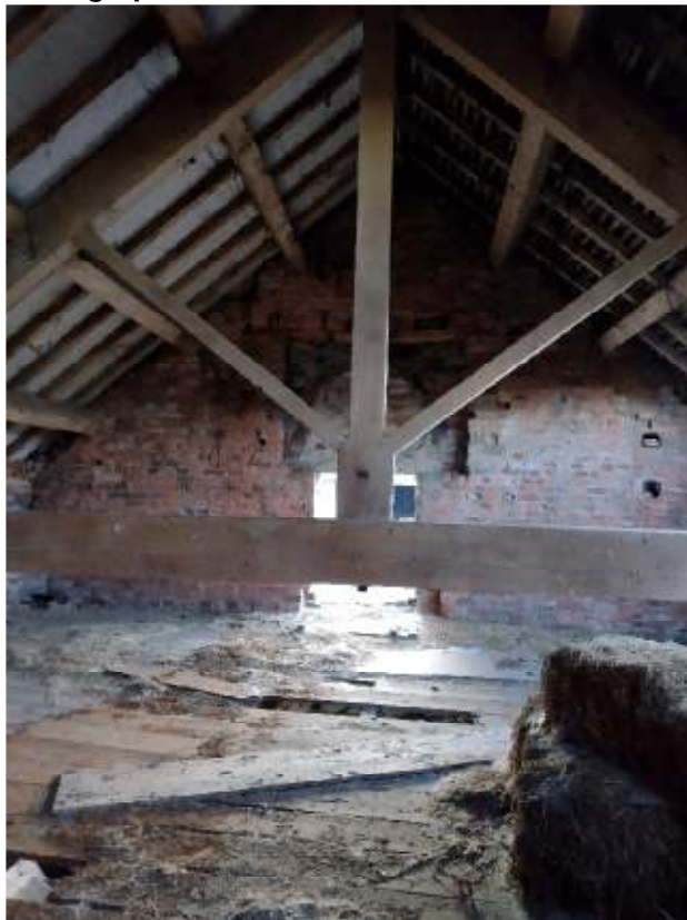
Photographic Plate 6: Internal view of first floor
