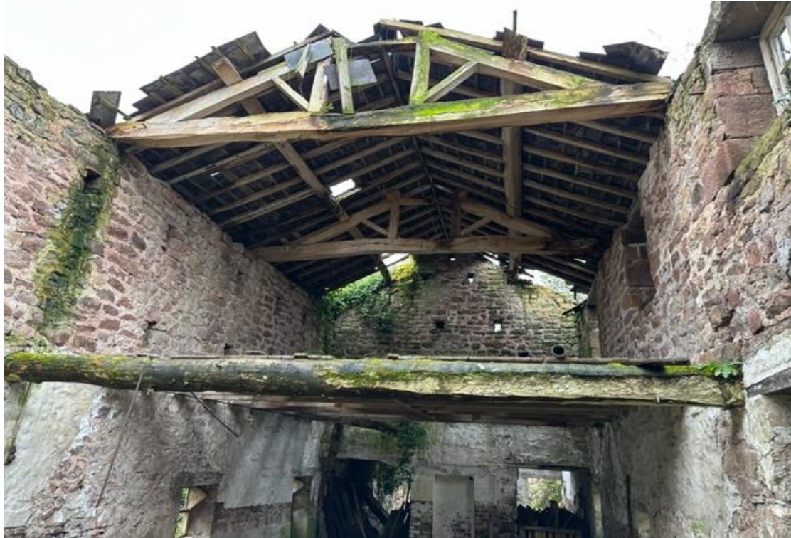
Typical internal view of southern wing of buildings – Stone work generally in good condition. Original remaining queen post trusses and purlins could be saved with minimal structural intervention.
