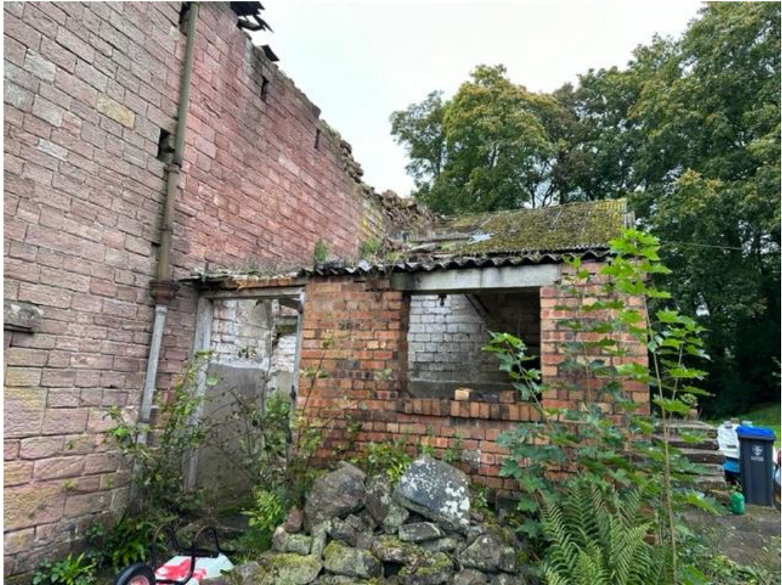
Small poor-quality brick-built structure to be demolished as part of the renovation.
