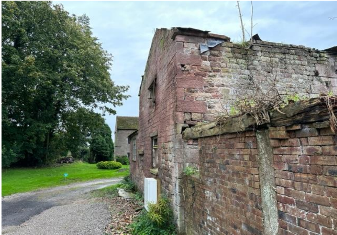
View of north east gable wall, cart shed in foreground and single storey outrigger in the background – note quality of stone work and plumb walls
