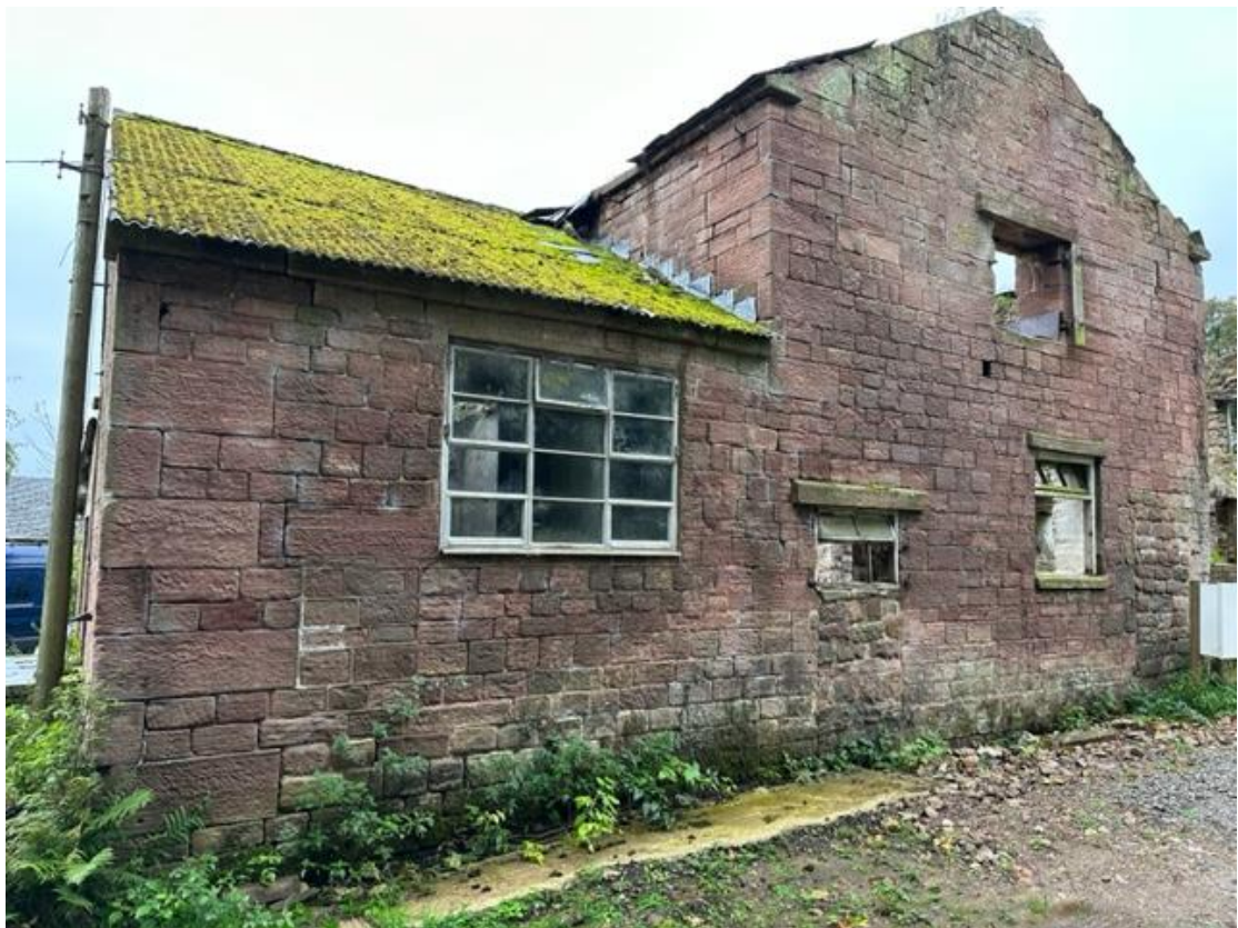
Further view of north east gable and single storey outrigger – note stone work in good condition and plumb, also note stone lintels in good condition.
