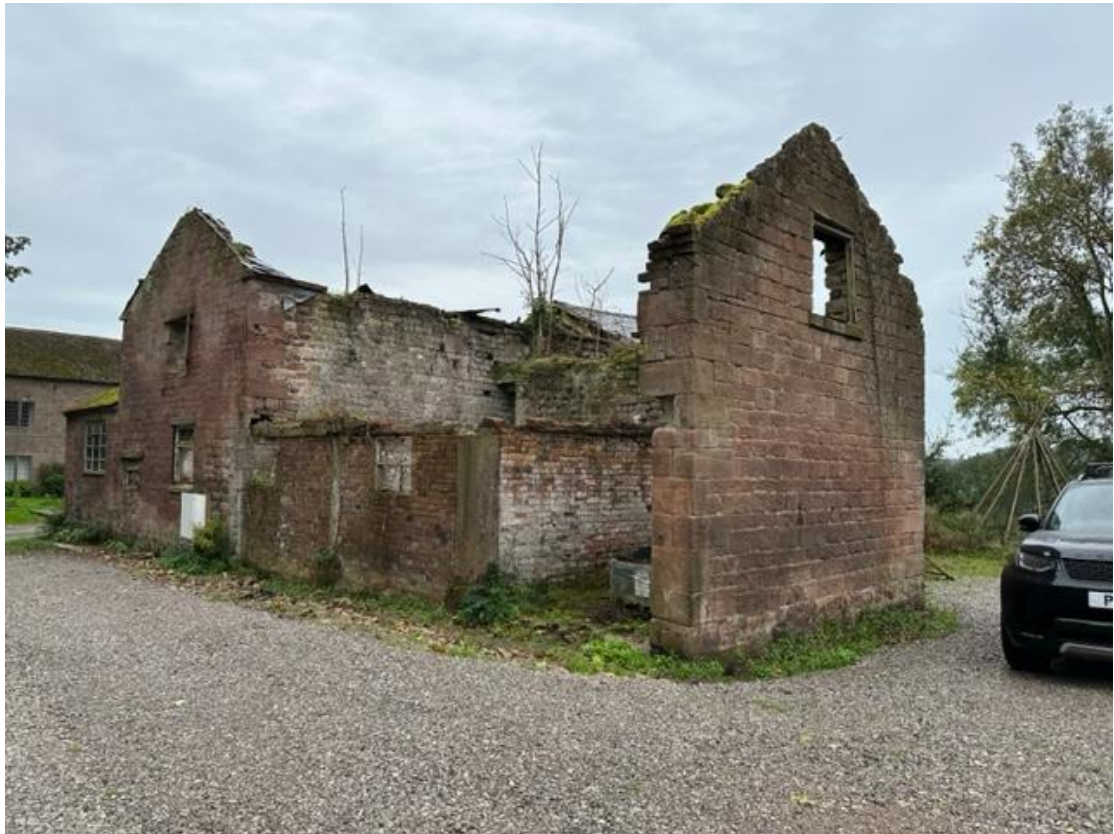
General view from North
