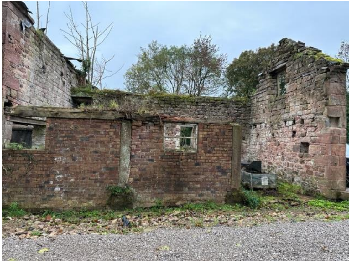
General view from the North east looking at the former cart shed – later brick infill panels with original stone pillars between.
