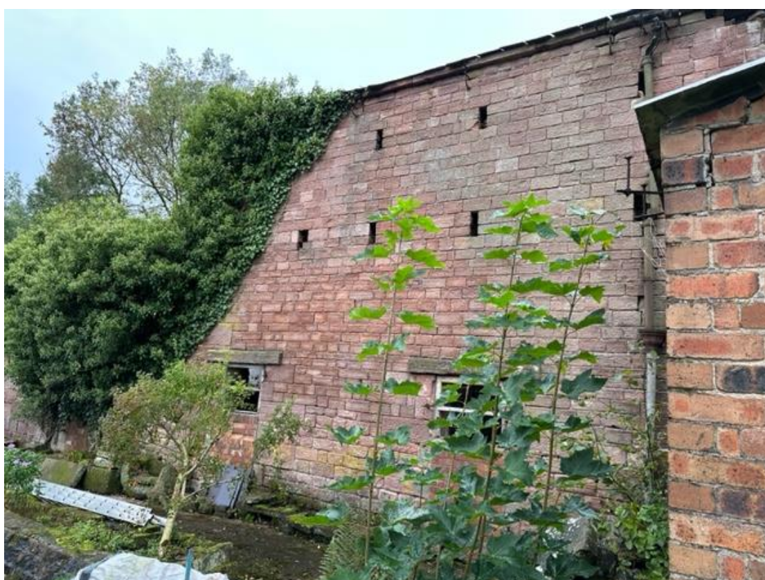
General view of south east elevation – stonework and lintels in good condition.
