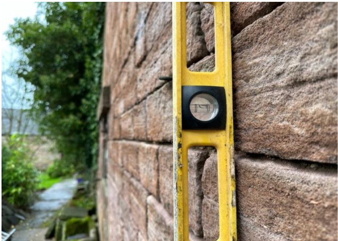
Close up of walls showing quality of stone and plumbness of walls
