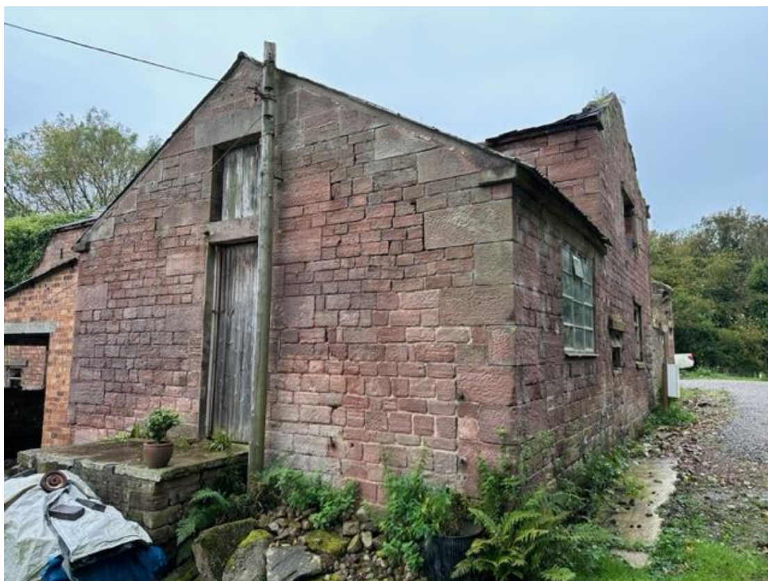
View of stone work to outrigger – Stone work in good condition and plumb.
