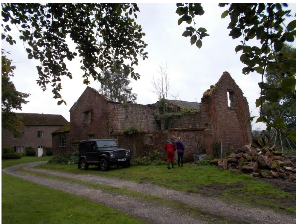
THE BARN VIEWED FROM THE NORTH WEST SHOWING THE ACCESS TRACK AND THE FARMHOUSE BEHIND TO THE LEFT
