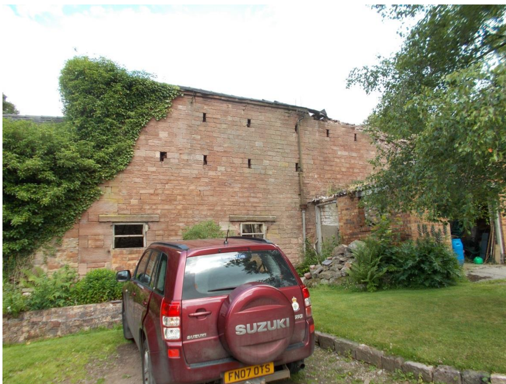
THE BARN FROM THE SOUTH EAST – SIDE FACING THE FARMHOUSE. Note fine quality of stonework
