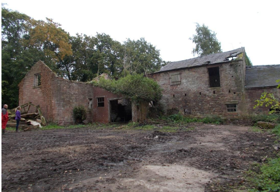
THE BARN FROM THE WEST
