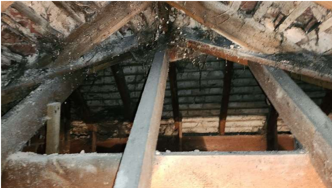
Plate 4: Showing internal roof void.
