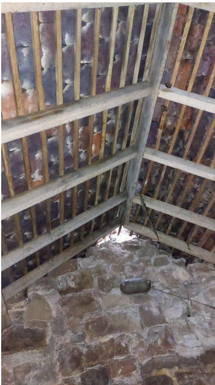
Plate 3: Internals of the structure with brown long-eared bats present
