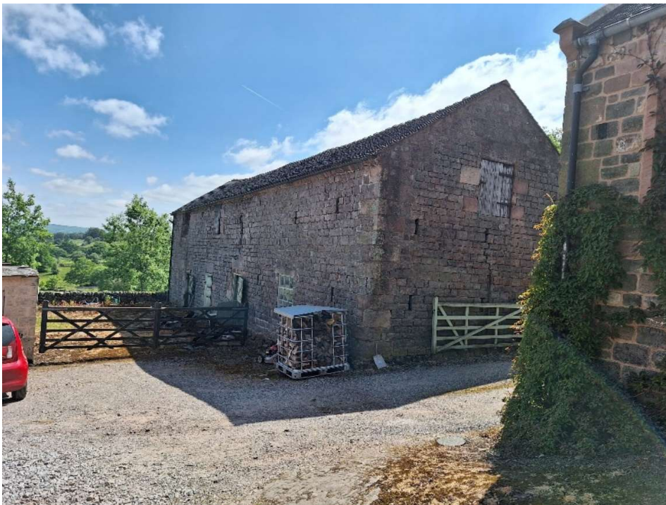
Photo 2 West gable elevation
