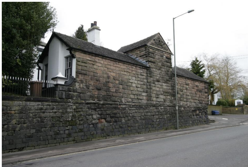
photograph 3 - view of the south and east elevations of the outbuilding
