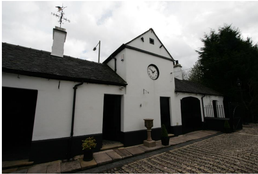
photograph 5 - view of part of the west elevation of the outbuilding
