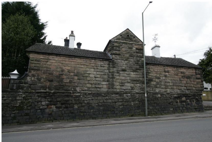
photograph 1 - view of the east elevation of the outbuilding
