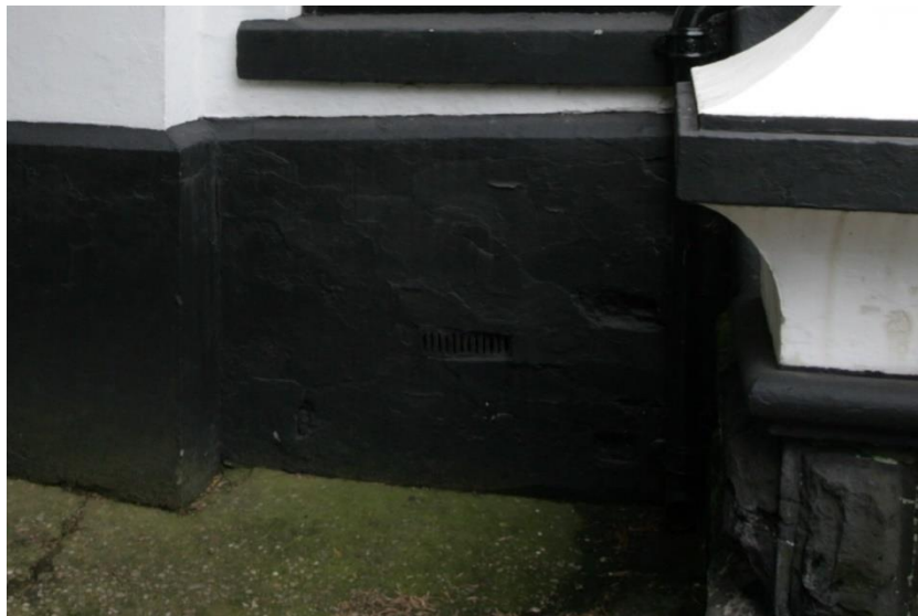
photograph 7 - view of one of the existing cast iron, hit and miss pattern, sub floor, air bricks this is on the south elevation
