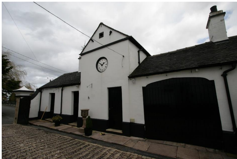
photograph 6 - view of part of the west elevation of the outbuilding
