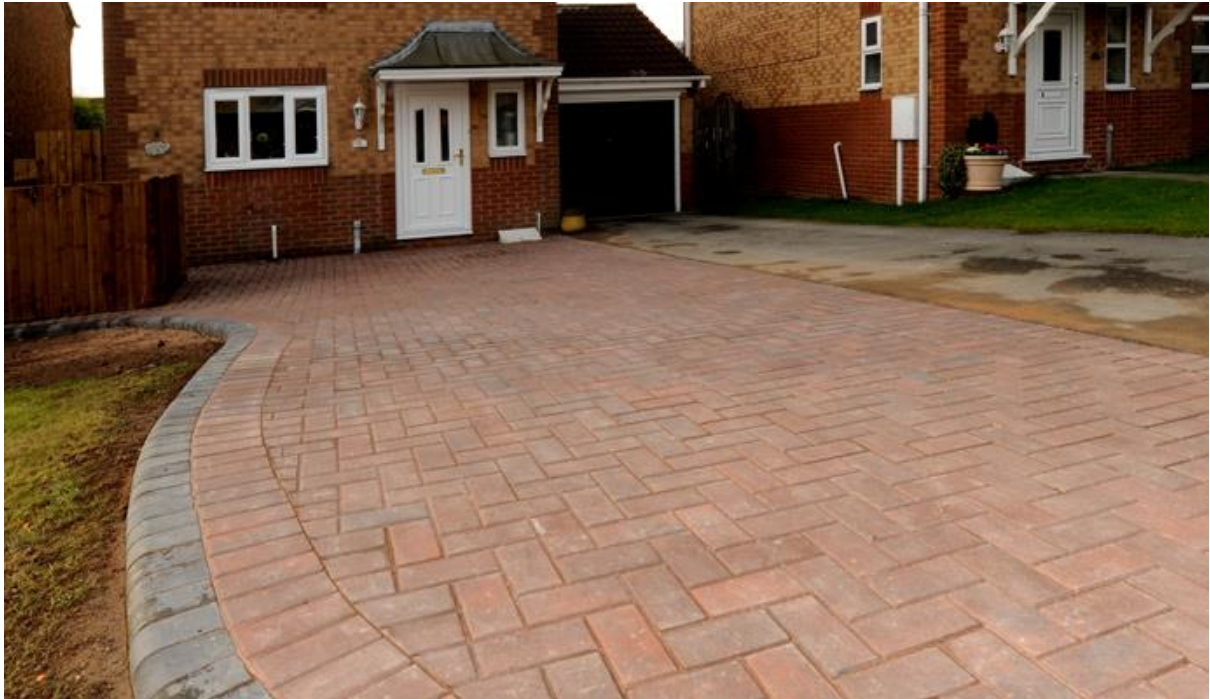
Hard Standing – Bradstone Block Paving
