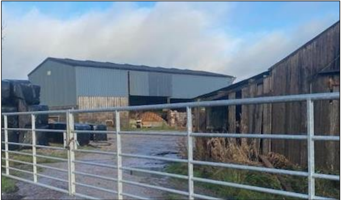
Figure 3 – Cladding at Little Paradise Farm
