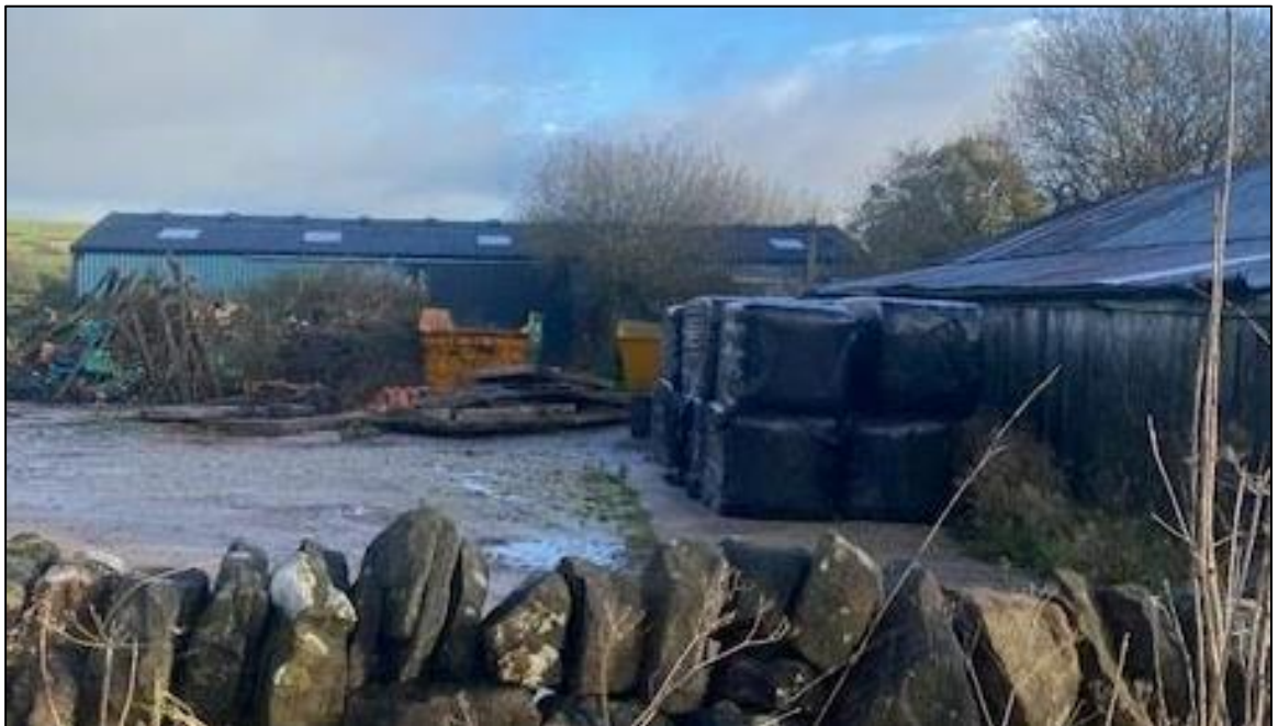
Figure 4 – Cladding at Little Paradise Farm
