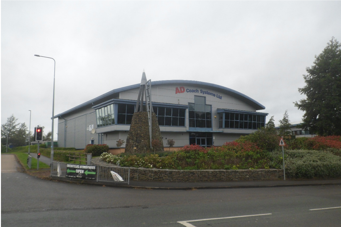
Plate 2 – Front elevation as viewed from the A527
