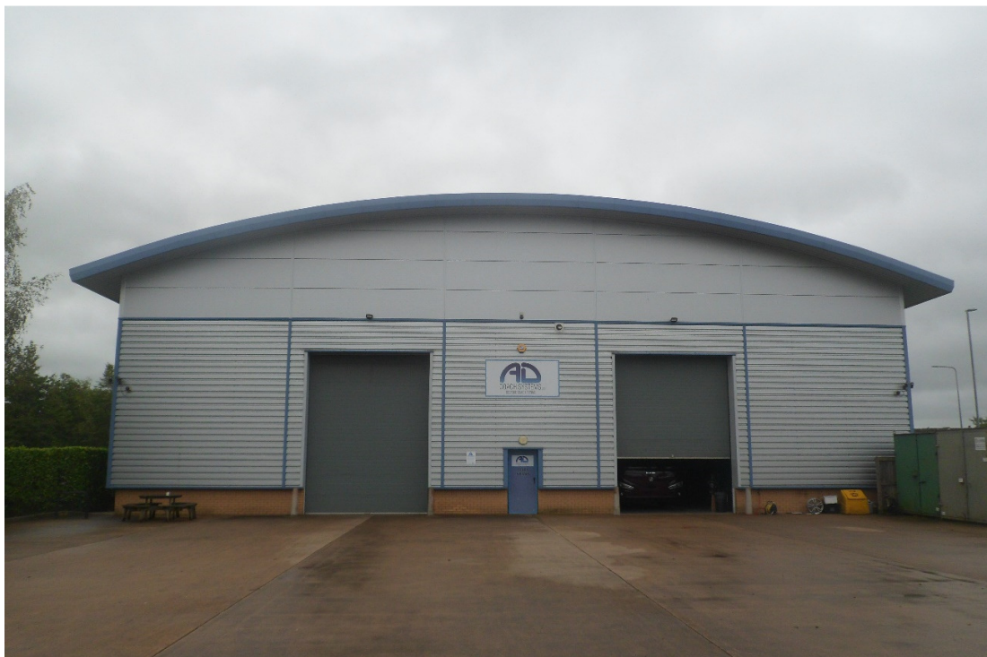
Plate 3 – Rear elevation looking East from the storage yard
