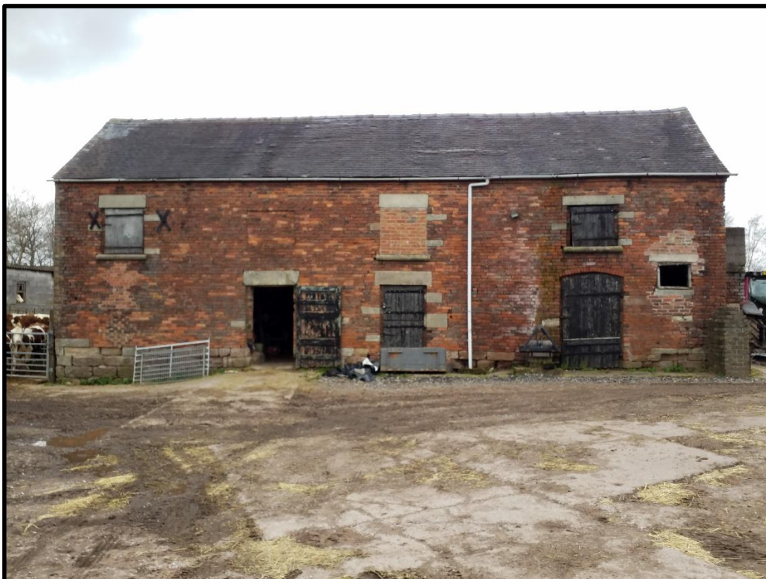
Photo 1 – shows the eastern elevation of the building.
