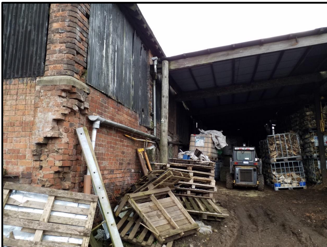
Photo 4 – shows part of the northern elevation of the building, including the 'lean-to' log store, which common pipistrelles were seen flying in and out of, in pursuit of prey.
