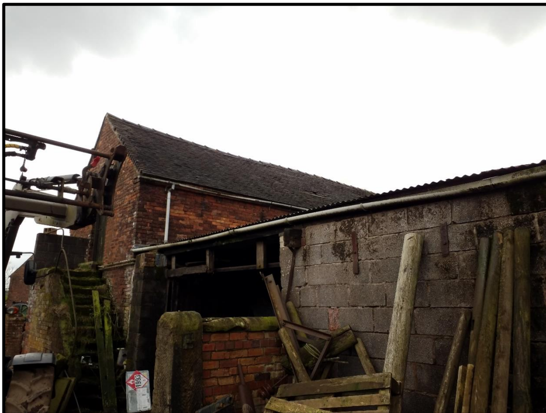
Photo 3 – shows part of the northern elevation of the building.
