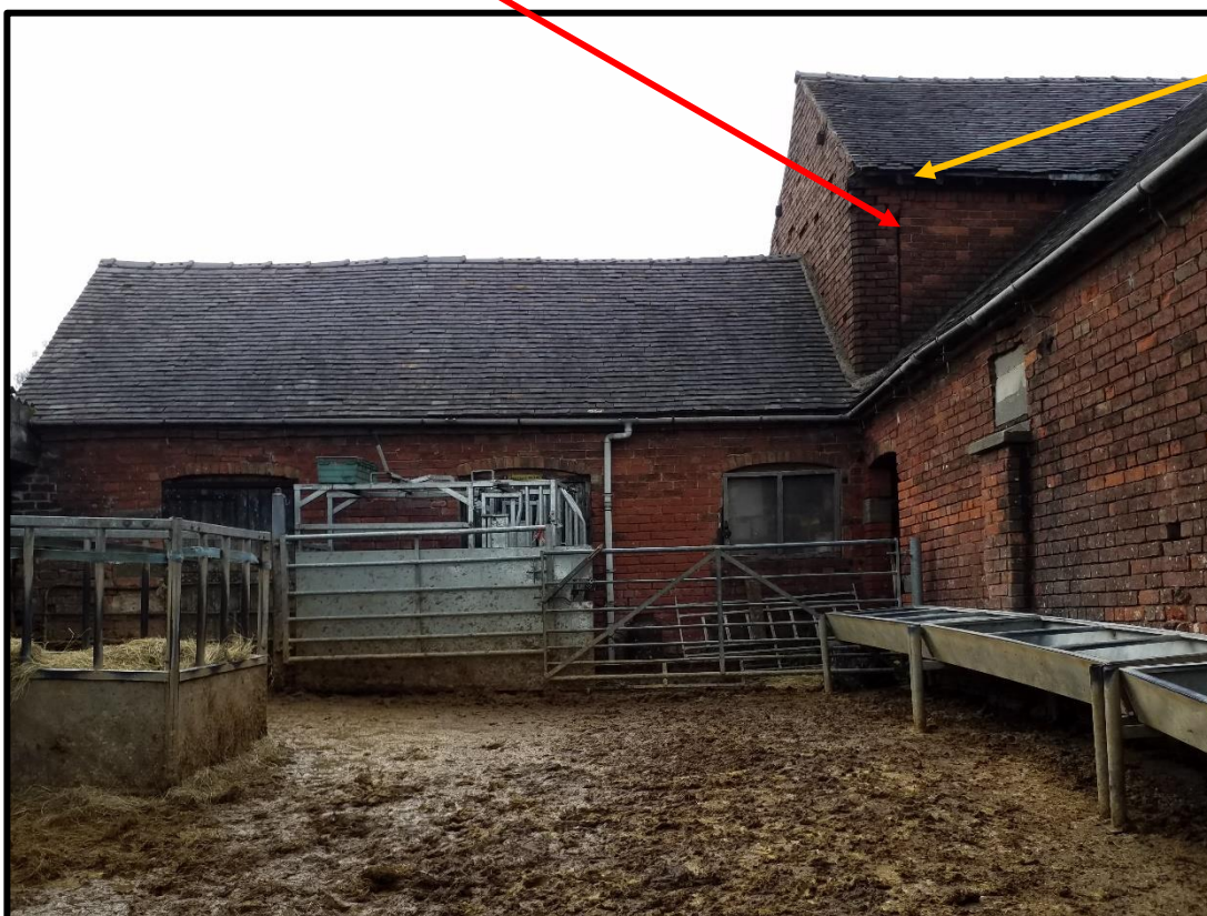
Photo 5 – shows the cattle yard and part of the south-western elevation of the building. The vertical crack and roof overhang where common pipistrelles were seen to emerge, are arrowed in red and orange respectively.
