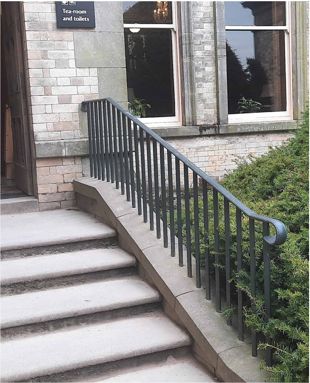
Existing guard-rail adjacent to tea room
