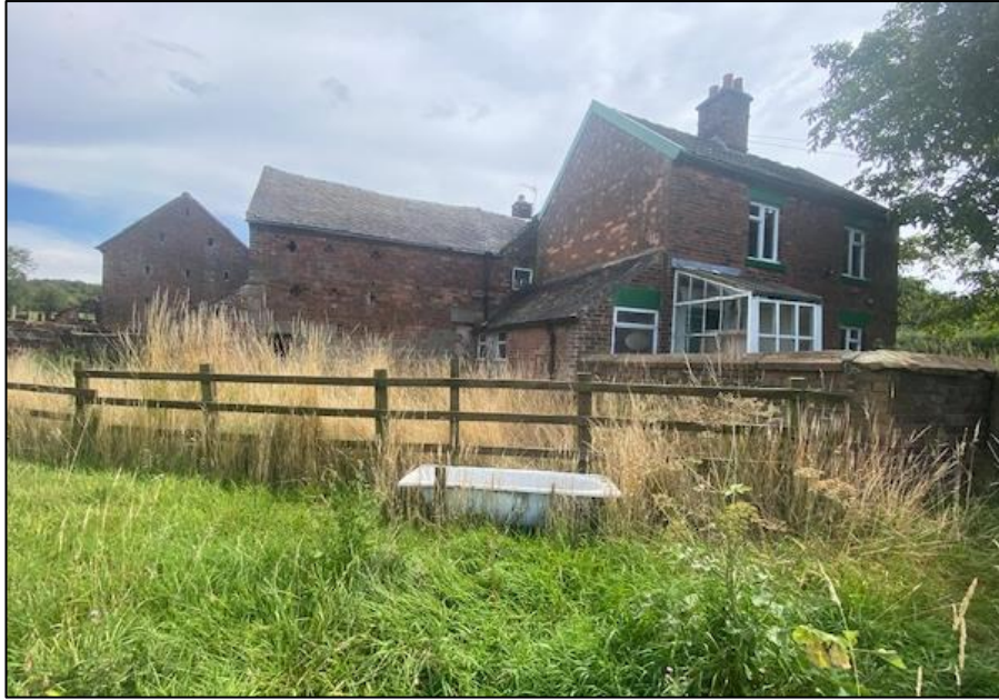
Plate 5: A photograph of the north and west elevations of the traditional barns and the farmhouse.
