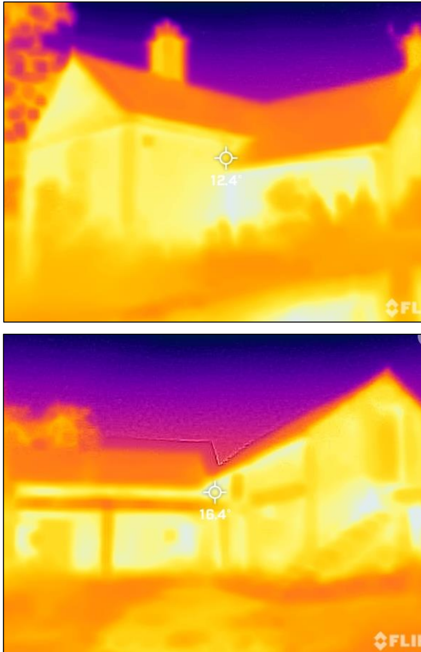
Figure 6 and 7: Thermal image of the farmhouse and the traditional barns
