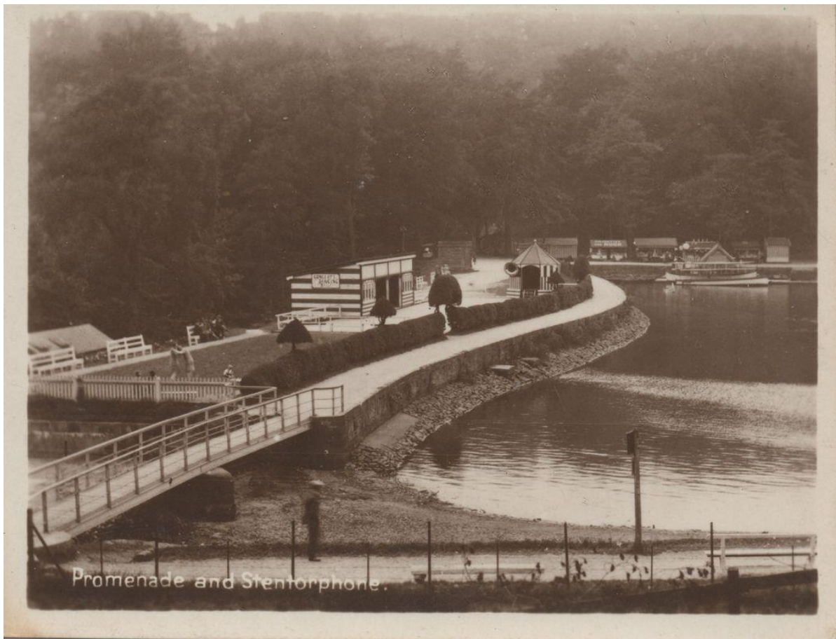
Figure 7: Photograph of Rudyard Lake dam, circa. 1920
