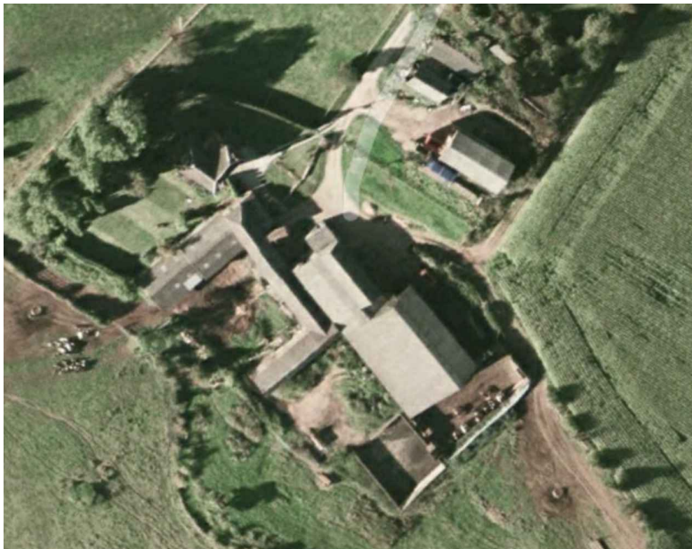
Original Site Aerial Photo Showing Extent of Barns NTS
