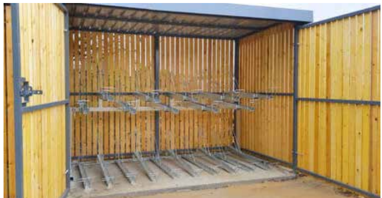
Figure 6: Internal view of typical two tier bicycle shelter.
