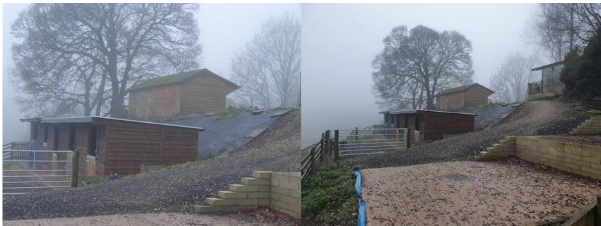
Existing stable block (background) in relation to concrete pads and extended track for intended stable blocks (foreground)
