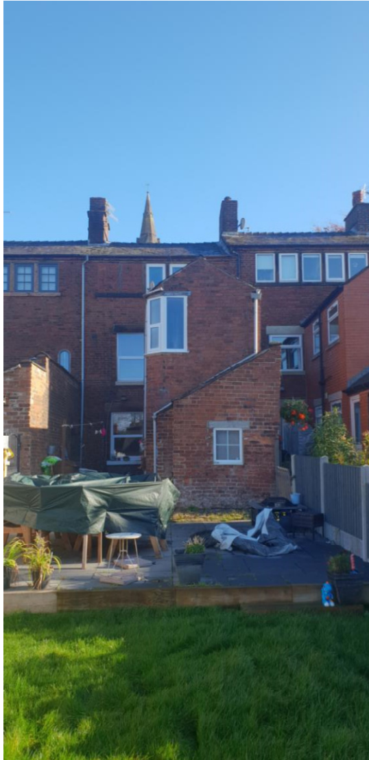
Rear of nr. 20 King Street
