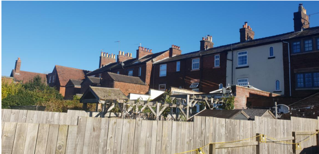
Neighbouring properties of 20 King Street, note blocked off weavers garret windows.
