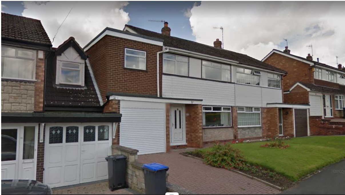
15 High view road 2 story flat roof extension
