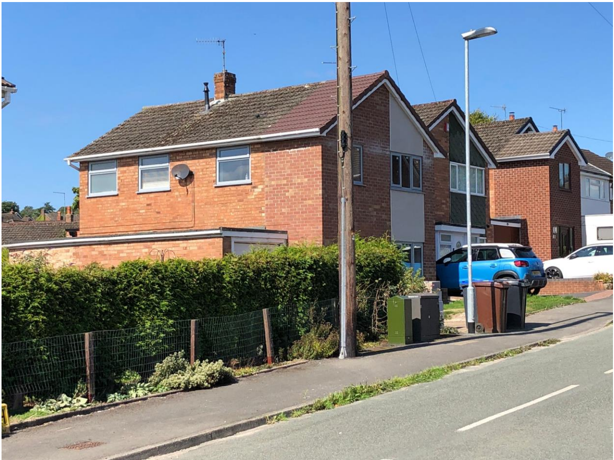
1 High View Road 2 story extension Visible from the road
