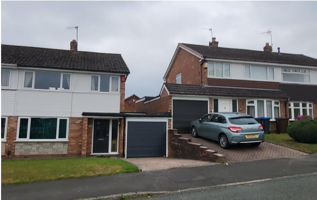
19 High View Road Tiered flat roof garage and extension
