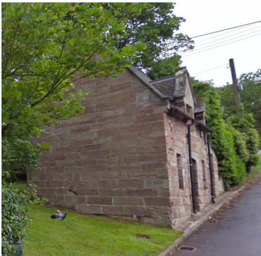
Log Store/Barn formerly cottage side elevation 2021
