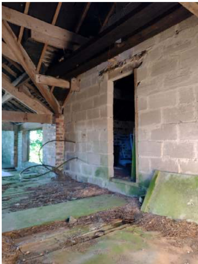
Photographic plate 4: Internal doorway which connects first floor sections
