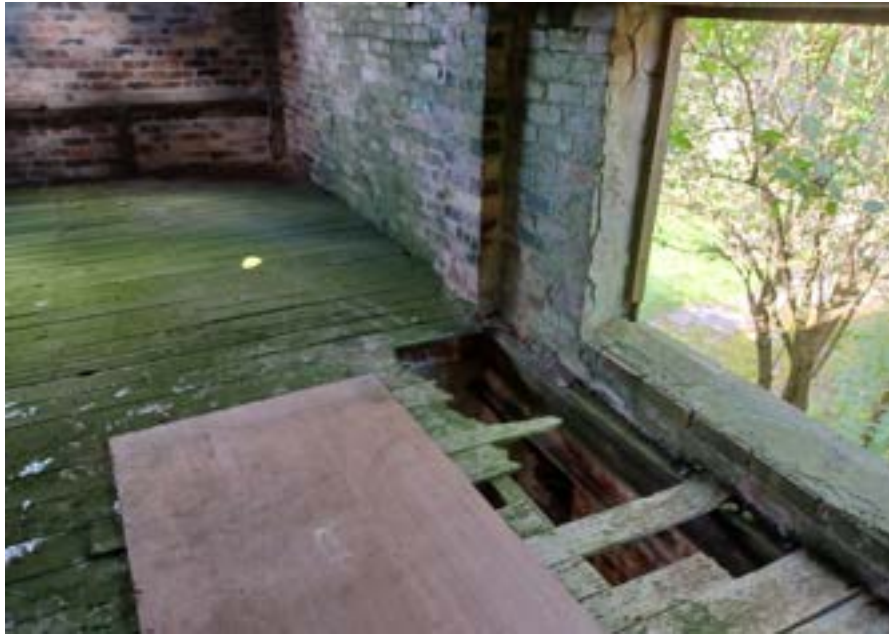
Photo 3 – Showing area of broken floor boards
