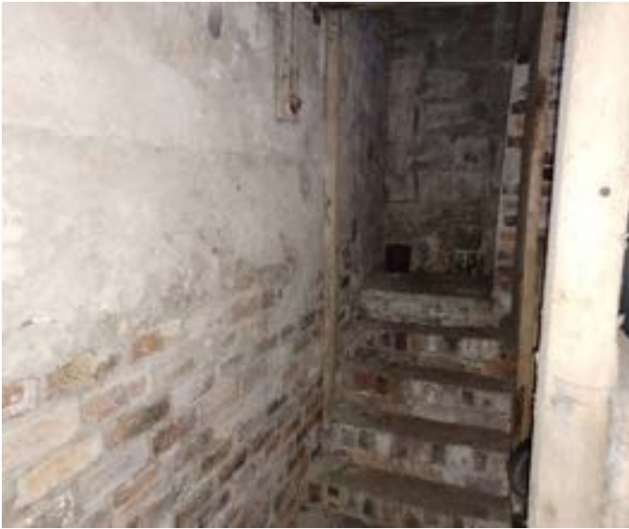
Photo 8&9 – 550mm brick external wall & internal stairs
