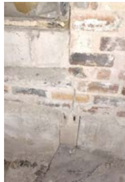
Photo 6 & 7 – Gable (retaining side) showing vertical crack below window
