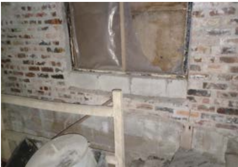
Photo 6 & 7 – Gable (retaining side) showing vertical crack below window
