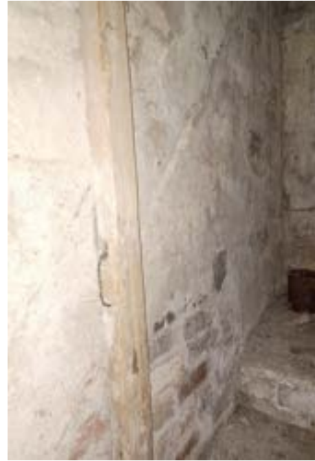
Photo 8&9 – 550mm brick external wall & internal stairs
