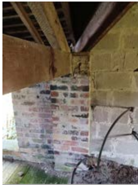
Photo 4 – Showing truss onto brick pillar
