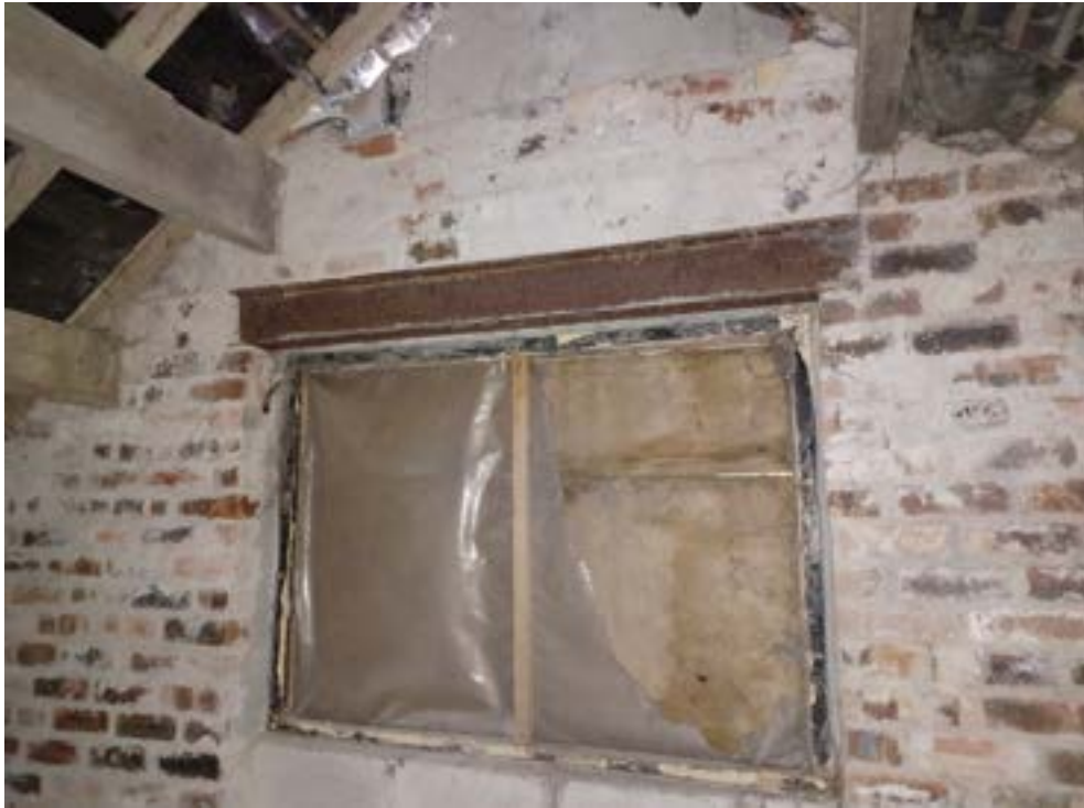
Photo 5 – Gable (retaining side) steel lintel to be treated
