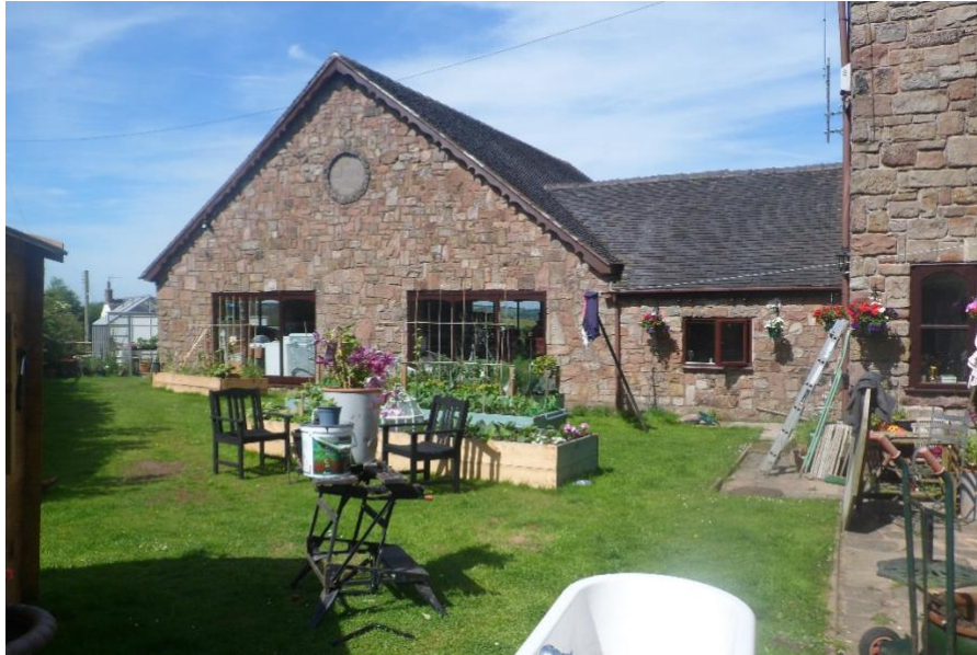
Image 4 – Front elevation of building to Hot Lane.
