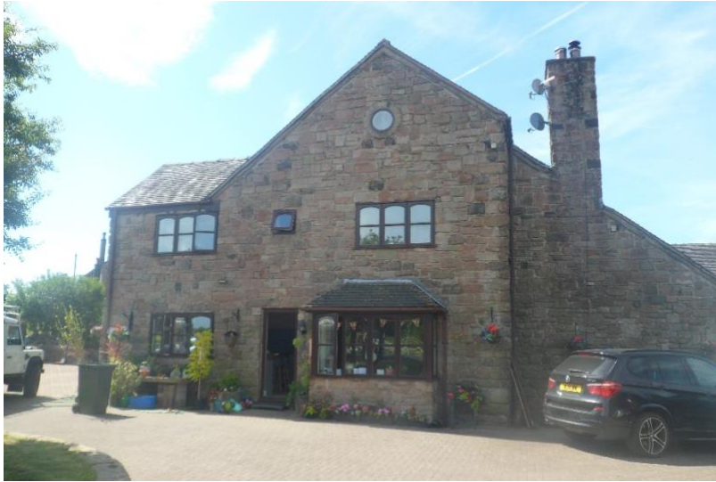
Image 2 – Main dwelling as viewed from Stanways Lane access point
