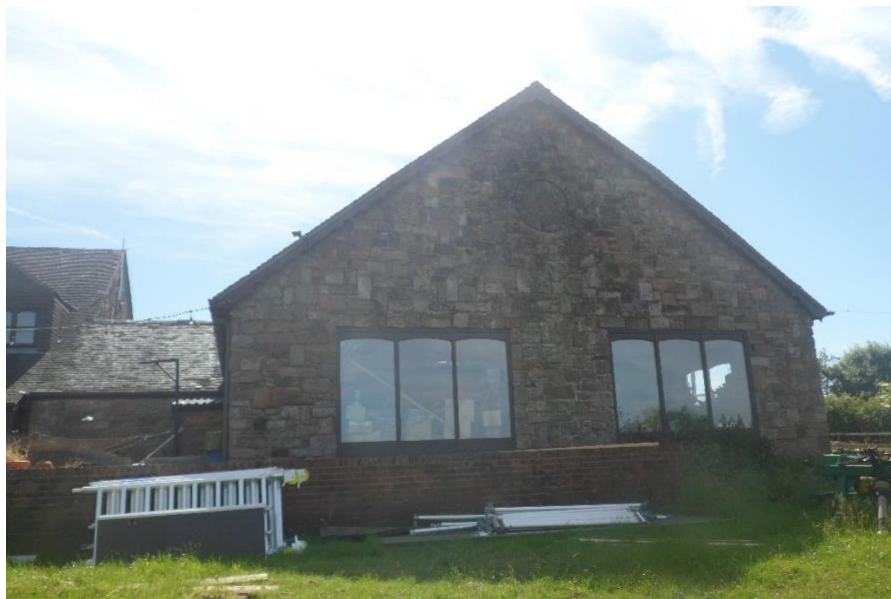
Image 5 – Rear elevation Facing North-West.
