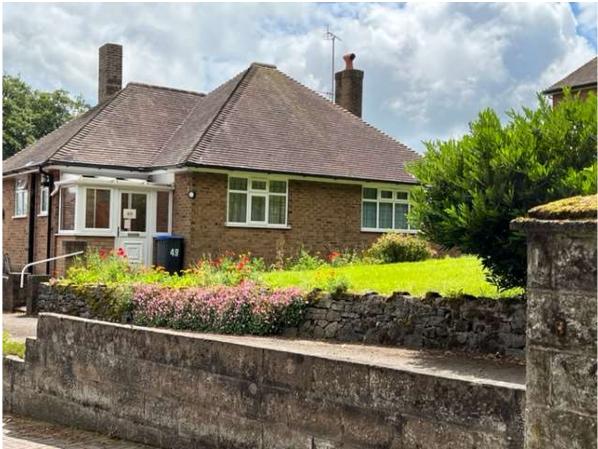
Number 47 is a simpler more linear bungalow constructed from a redder facing brick, darker roof tile, brown window and projecting bay window.
