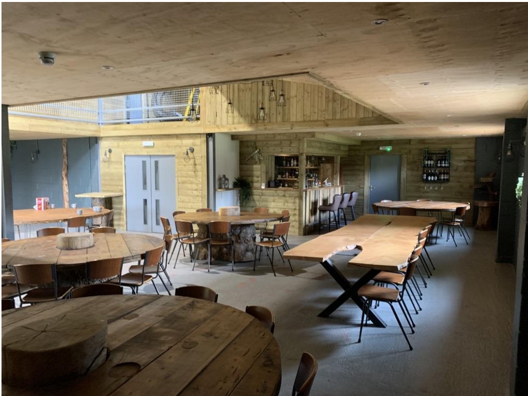
Figure 2: Image of venue post to remedial works.
