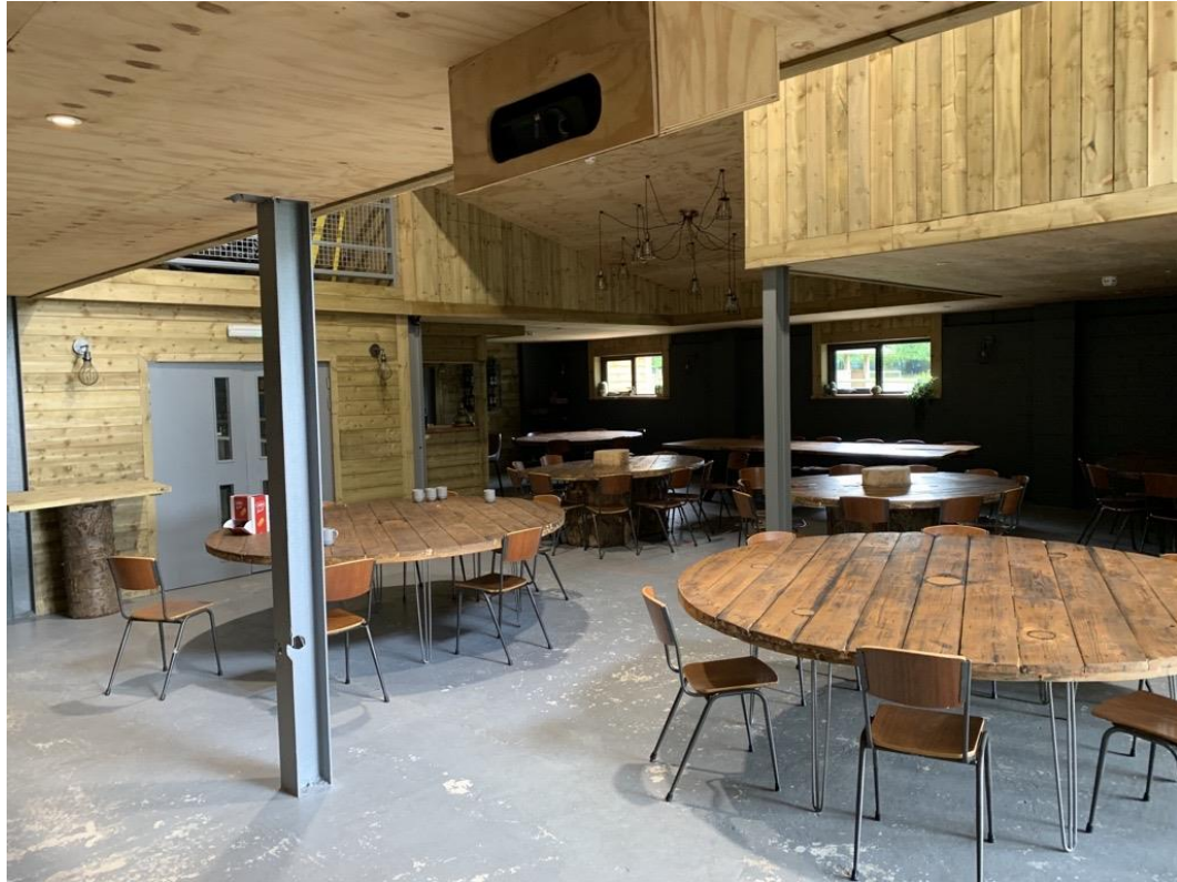
Figure 3: Image of venue post to remedial works.
