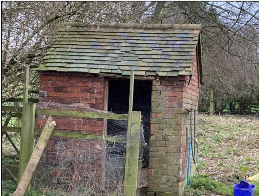
Photograph 10 showing the brick-built shed
