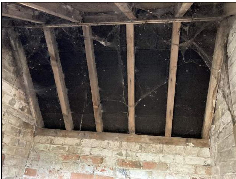
Photograph 11 showing the inside of the shed
