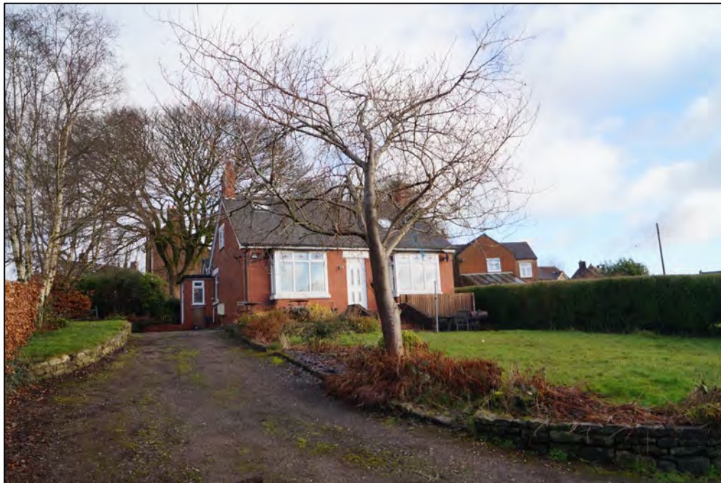
Plate 1. Looking northwards from the bottom of the PDA.
