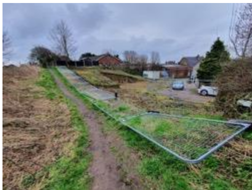
Figure 9. Footpath adjacent to northern boundary.
