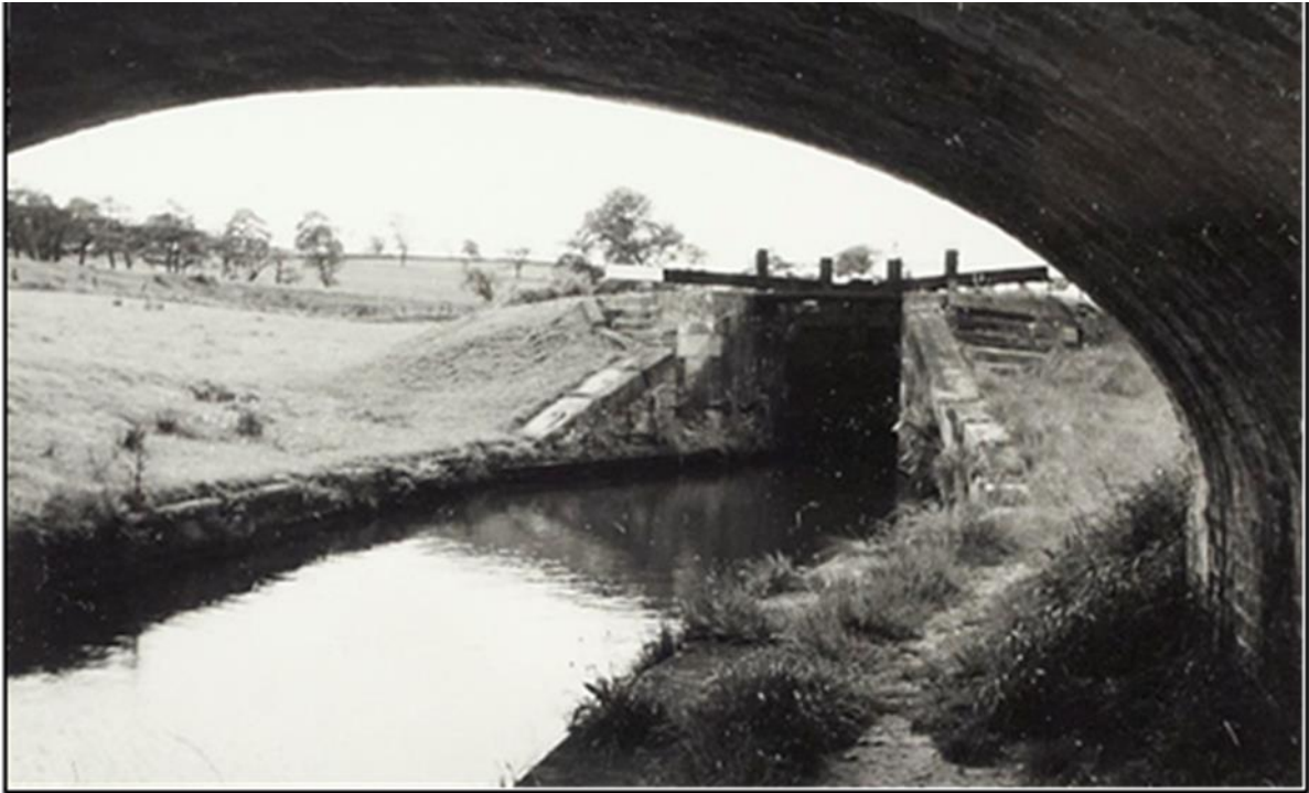
Figure 1: The underside of Bridge 37 looking towards Hazlehurst Lock 12 circa 1962 (Canal & River Trust Archives). This demonstrates the close relationship to Lock 12 and how Bridge 37 has an impact on the setting of Lock 12.
