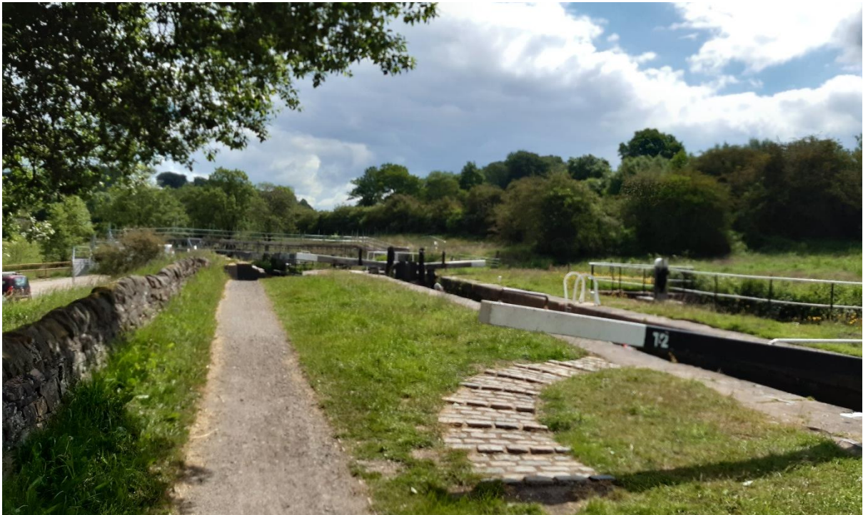
Figure 9: Lock 12 looking towards where Bridge 37 stood, the remains of towpath abutment can be seen.
