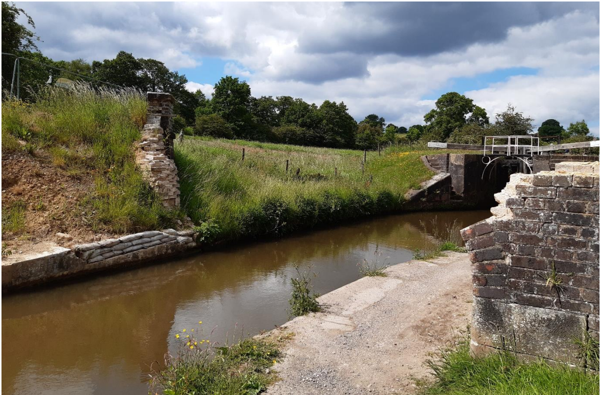
Figure 10: The remains of the offside and towpath abutment of Bridge 37 after the partial demolition. Lock 12 is designated and had group value with the bridge.
