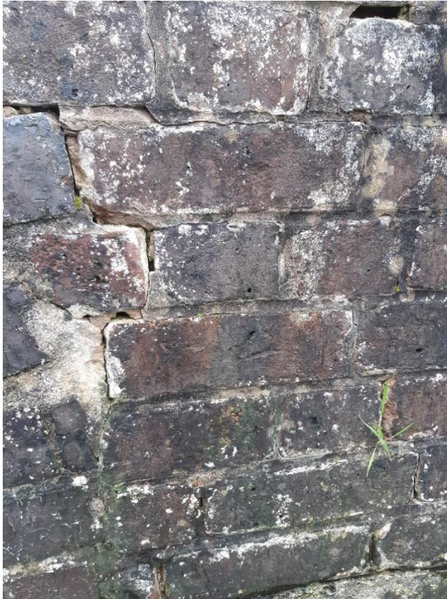
Figure 3: The bricks at bridge 37.
