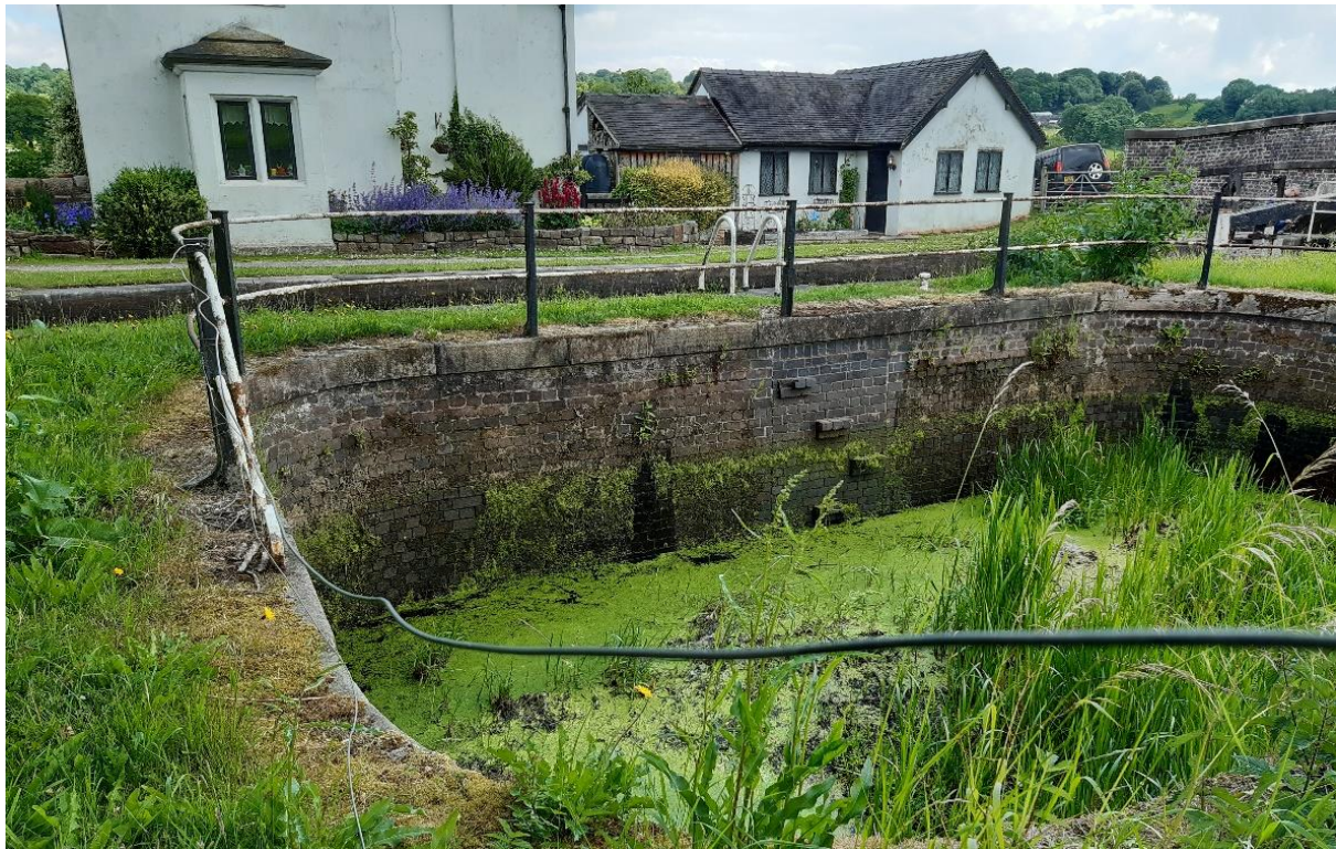
Figure 7: Weir at Hazlehurst Junction.
