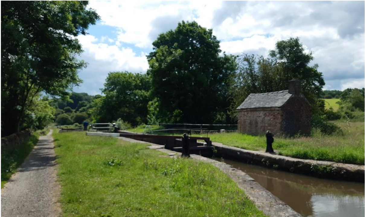
Figure 8: Lock 11 with hovel part of the rich canal scape at Hazlehurst lock flight. Lock 12 and Bridge 37 are just beyond.
