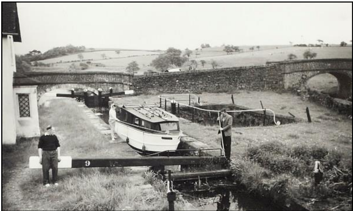
Figure 2: Hazlehurst Junction circa 1962 (Canal & River Trust archives).
