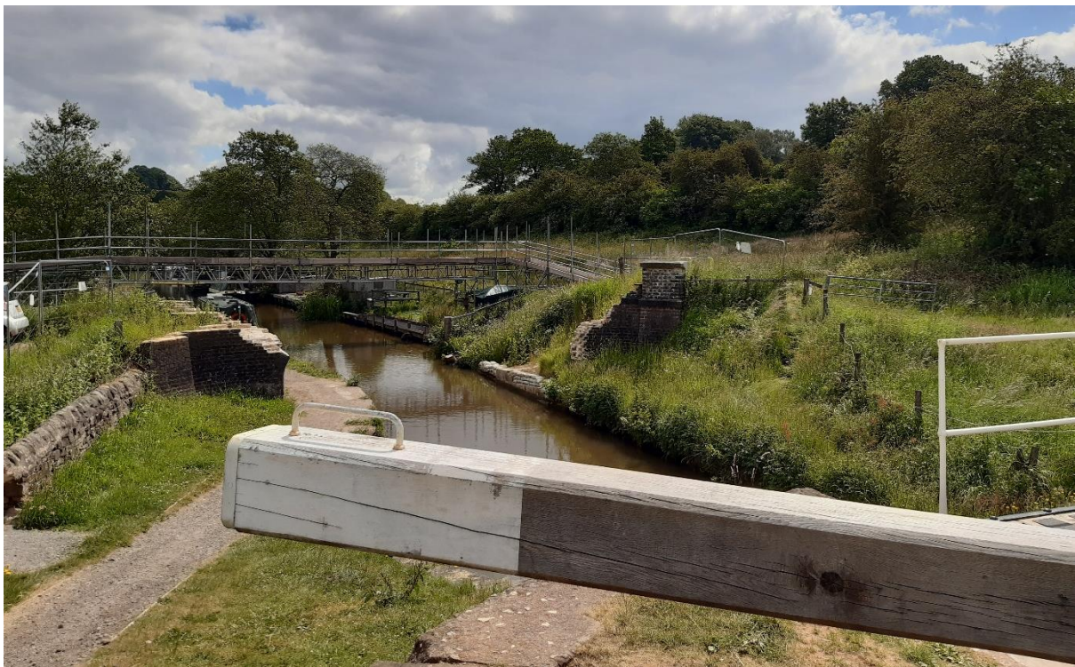
Figure 4: The view from Lock 12 with the remains of Bridge 37 in the background.
