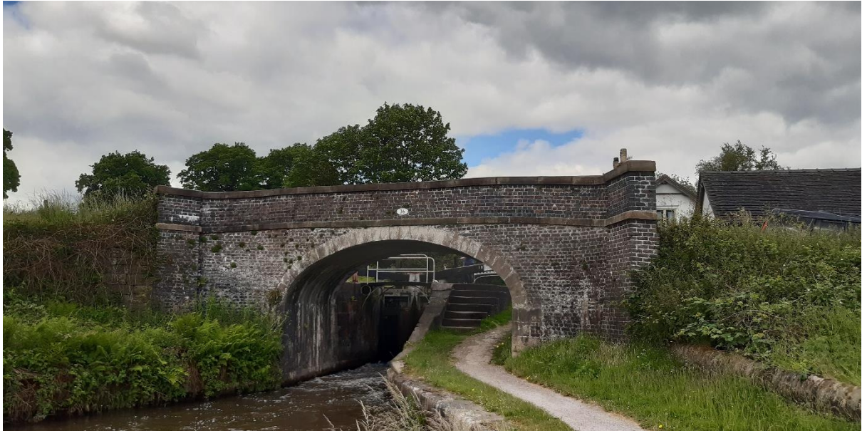
Figure 6: Bridge 36 is a similar design and constructed from the same materials as at Bridge 37. Bridge 36 and 37 were both designed by John Rennie.
