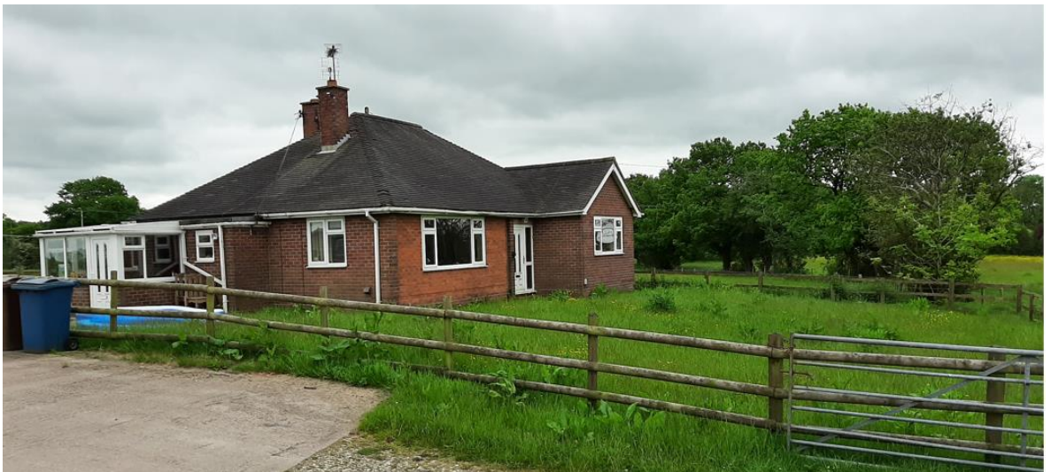
Plate Two: Photograph of the property as purchased by the applicant.
